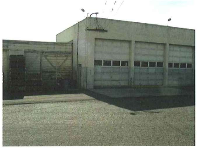
Photograph 8. Former truck maintenance building on the WHC Property. Photo facing south.
