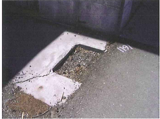
Photograph 10. Dispenser island footprint adjoining the former truck maintenance facility on the WHC Property.
