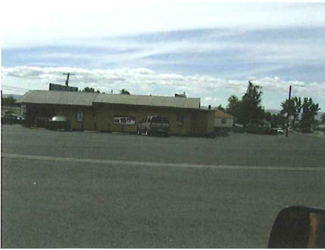
Photograph 1. The Property's convenience store building with South First Street in the foreground.
