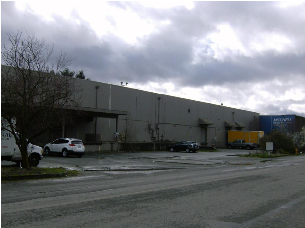
Photo 4: West Side – from the southwest
