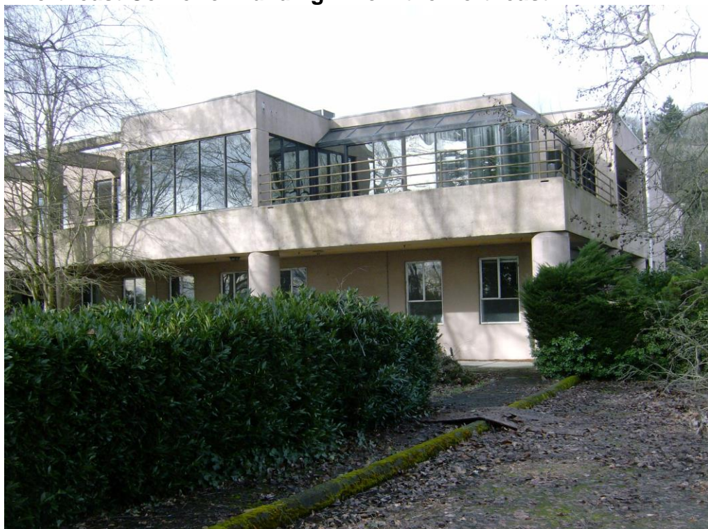
Photo 2: Northeast Corner of Building – from the Northeast
