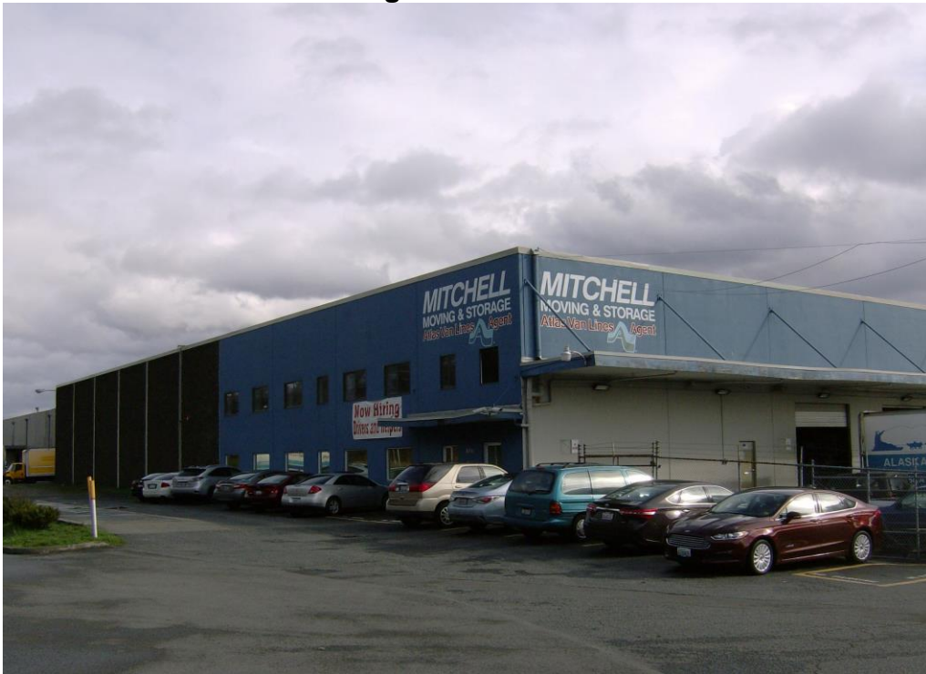
Photo 1: Southwest Side of Building - from the southwest
