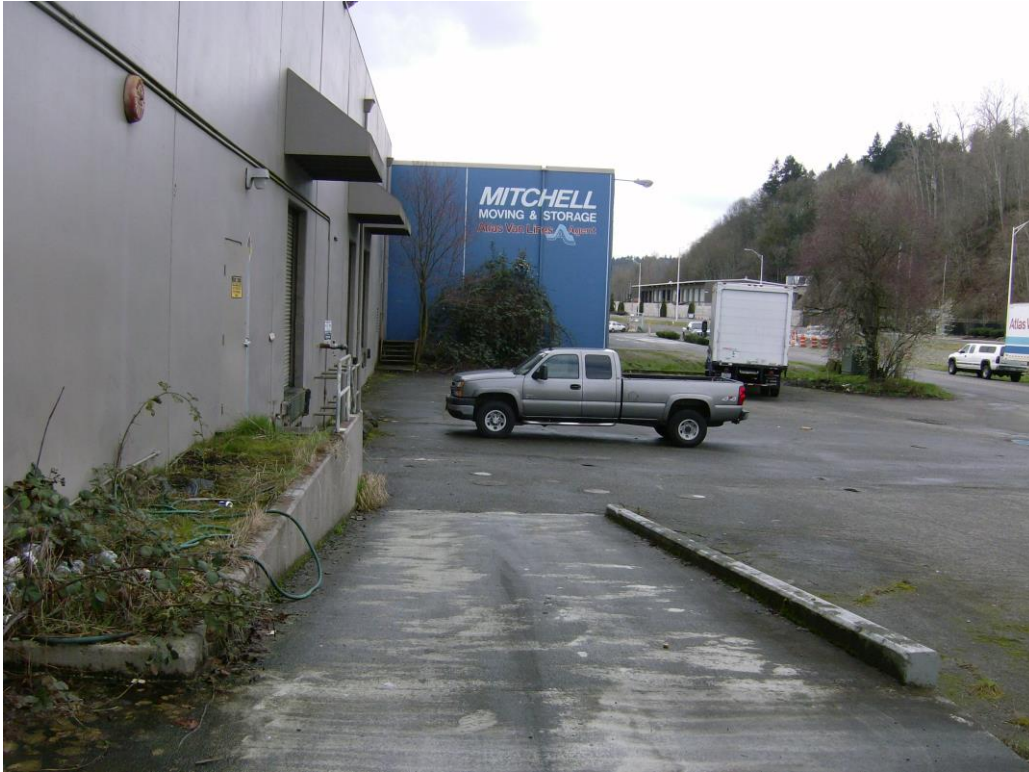
Photo 3: Former Tank Area – from the north.
