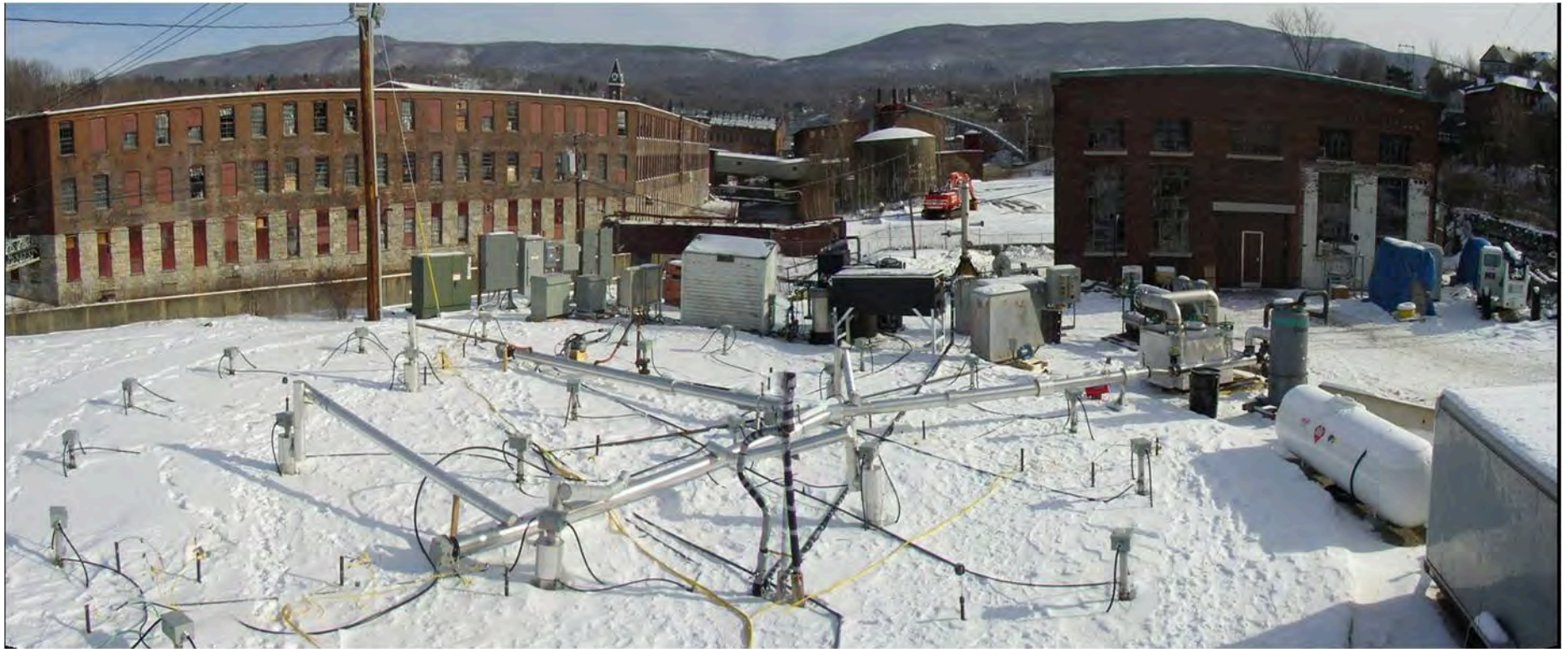
Note: Photograph provided by R. Baker, TerraTherm, Inc.
