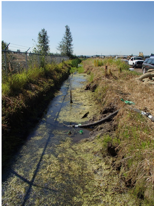
Photograph 2. Water diversion in the South Ditch
