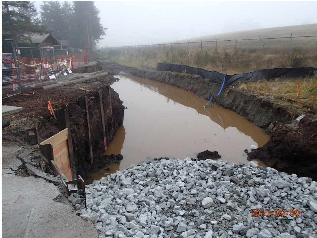
Photograph 15. Quarry spill in South Ditch excavation
