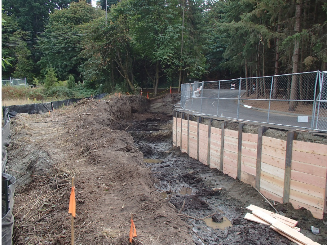
Photograph 13. South Ditch excavation and shoring
