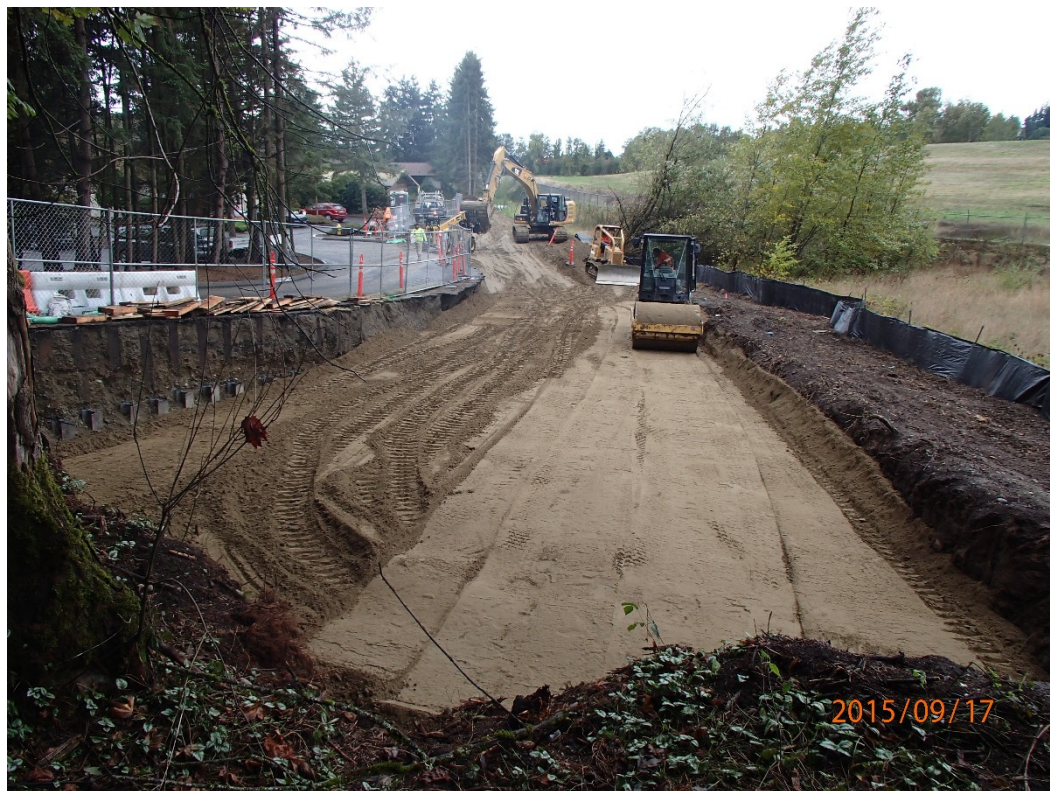
Photograph 19. Backfill and compaction in the South Ditch
