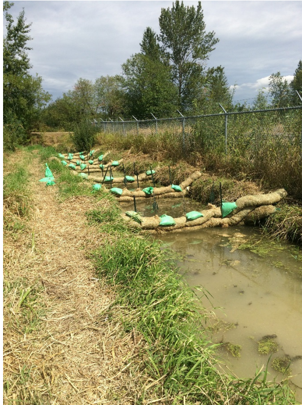
Photograph 5. Straw wattle dams in the South Ditch
