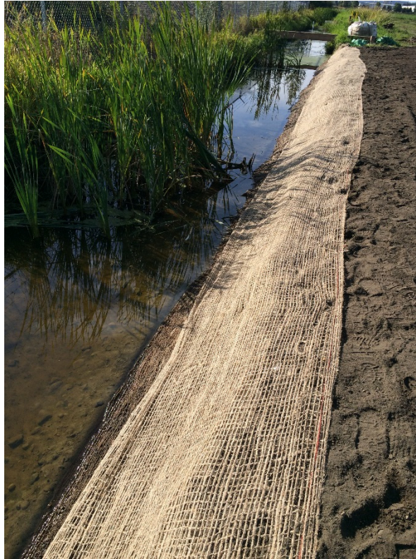
Photograph 7. Jute mat in the West Ditch
