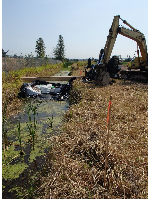
Photograph 1. Upgradient check dam in the South Ditch
