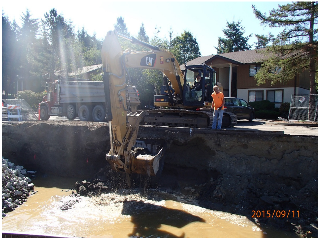
Photograph 16. Over-excavation on the South Wall between CP-10 and CP-12
