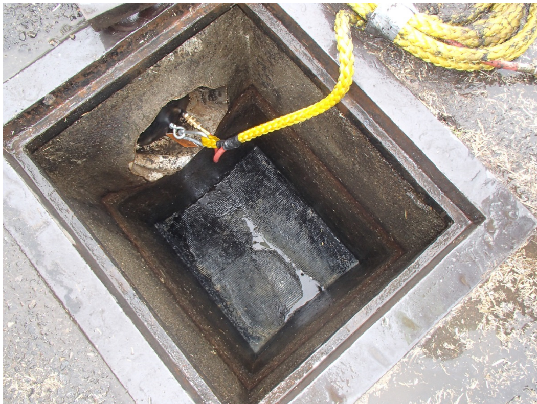
Photograph 18. Installed catch basin plug
