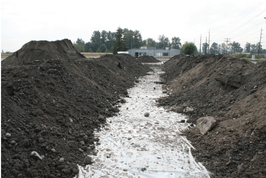
15. View of the dip tank area waste soil in windrows for characterization.
