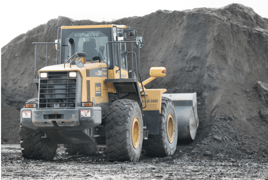
14. View of the front end loader moving the stockpiled waste soil into windrows.
