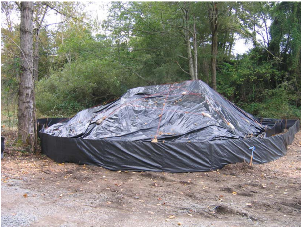
Stockpile covered with surrounding silt fence.
