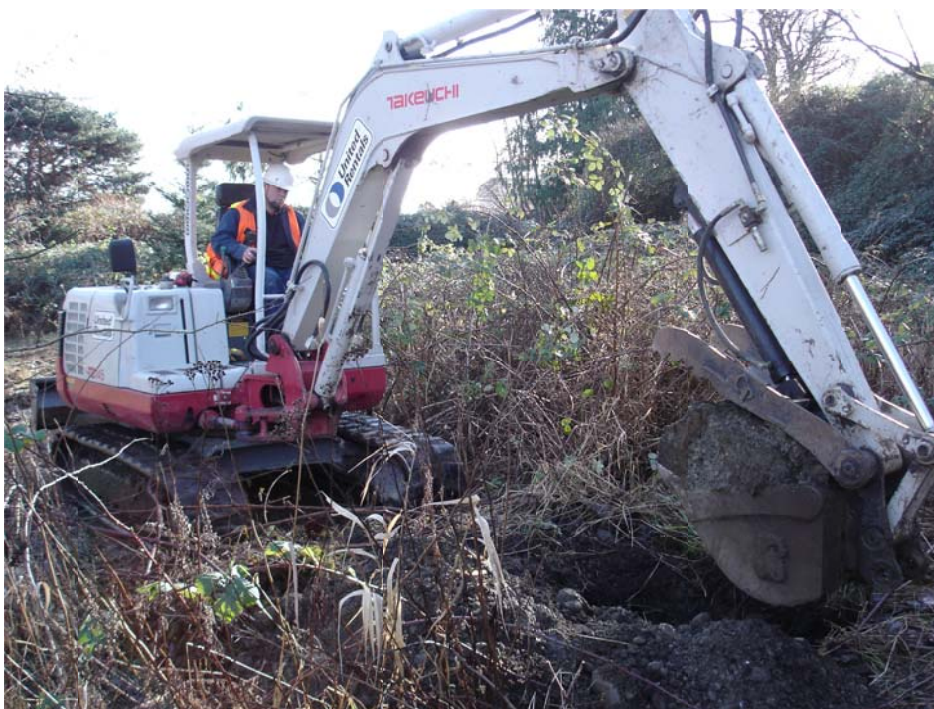
Small track excavator used to excavate test pits. Reconnaissance test pit RTP-13 is shown in the photo.
