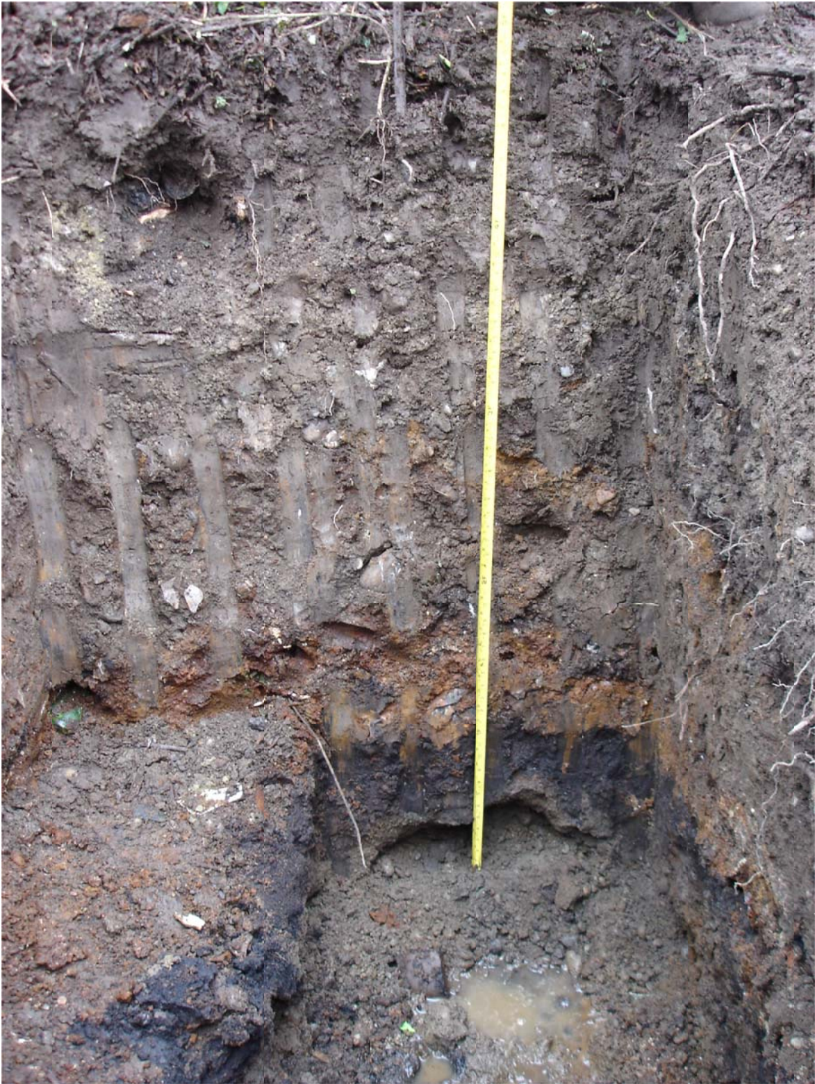
TP-23 South Sidewall at 5 ft bgs
