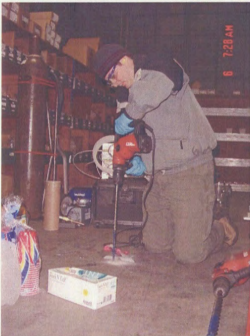
Sub-slab Sample Location V-1 – Drilling Sample Probe Location
