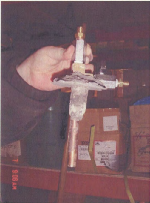
Sub-slab Sampling Probe (after removed from a sample location)
