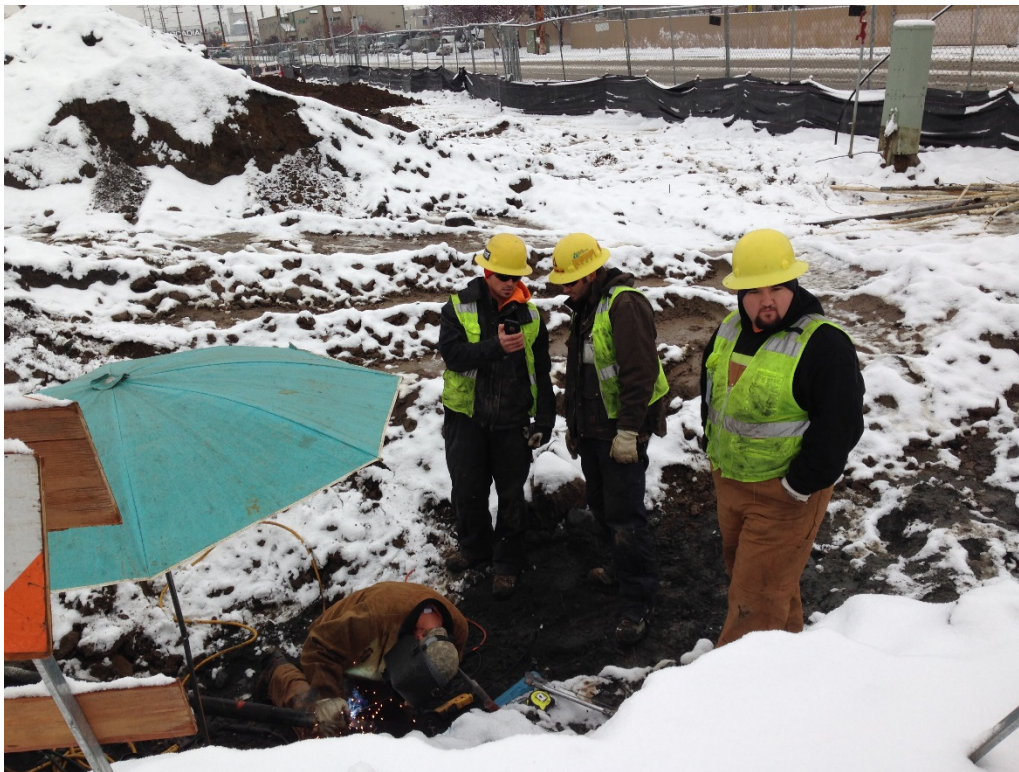
Figure 6: Cascade Natural Gas Co. Natural Gas Line Capping (12/03/2015)
