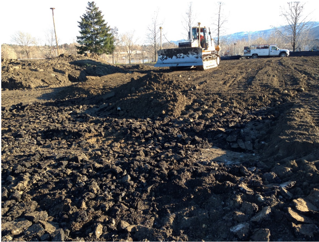
Figure 7: Rubbleized Asphalt (12/14/2015)
