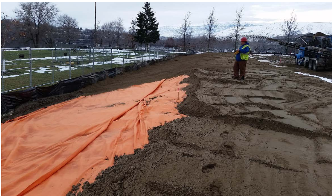
Figure 10: Cap Construction— Topsoil (01/26/2016)
