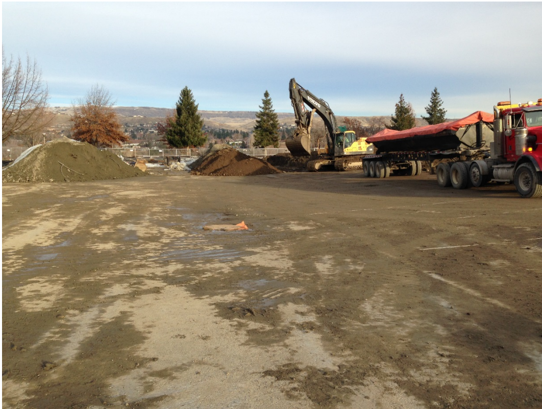
Figure 9: Refuse Loading for Off- Site Disposal (12/15/2015)
