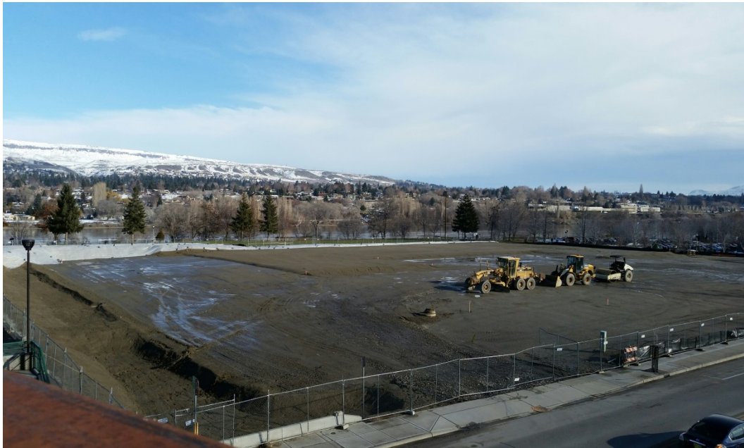
Figure 11: Post Cap Construction (01/31/2016)
