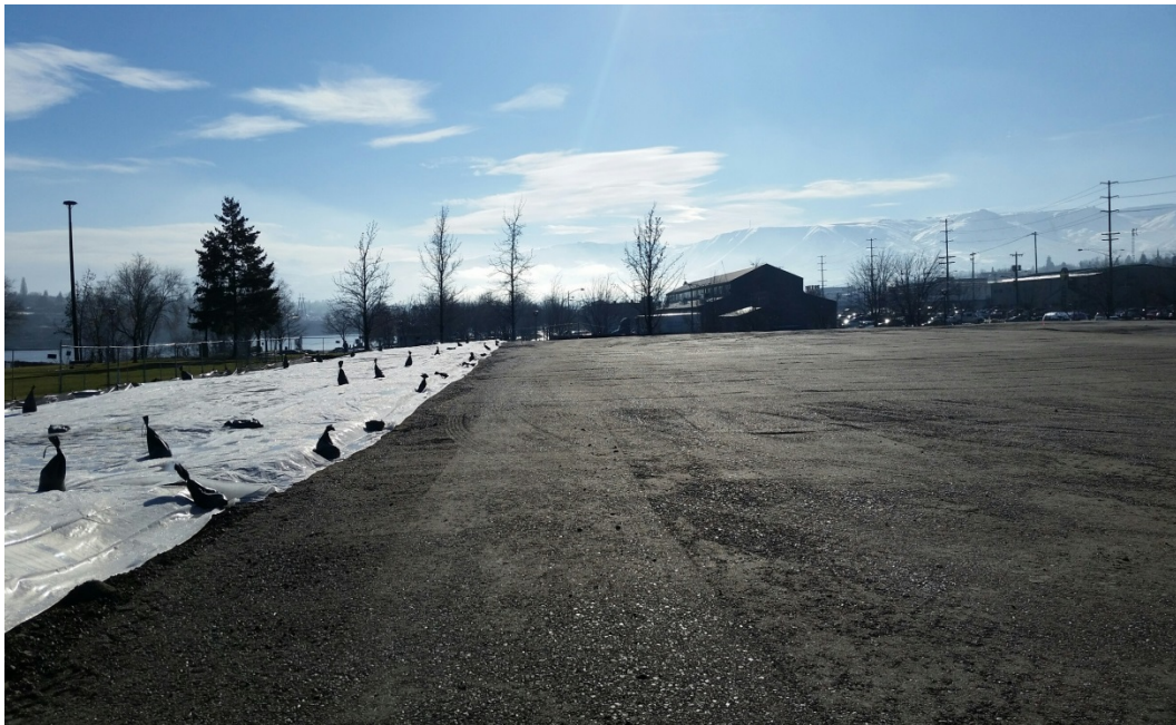
Figure 12: Post Cap Construction— Topsoil Covered with Plastic Sheetting (01/31/2016)
