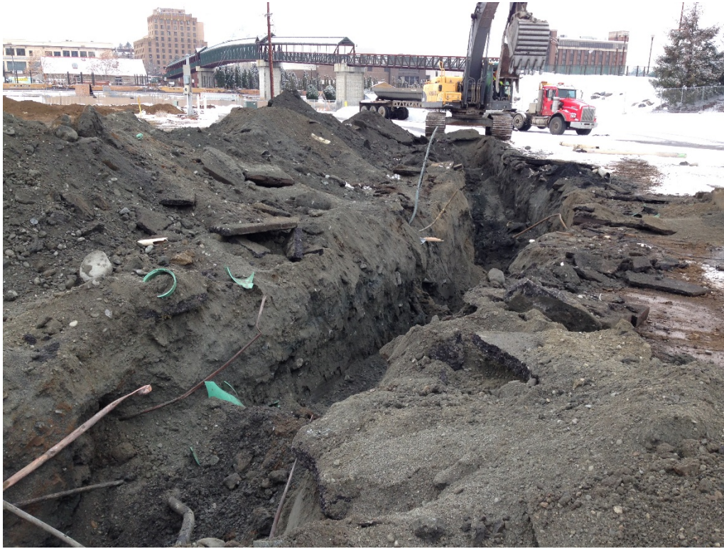
Figure 3: Sanitary Sewer Line Demolition (12/02/2015)
