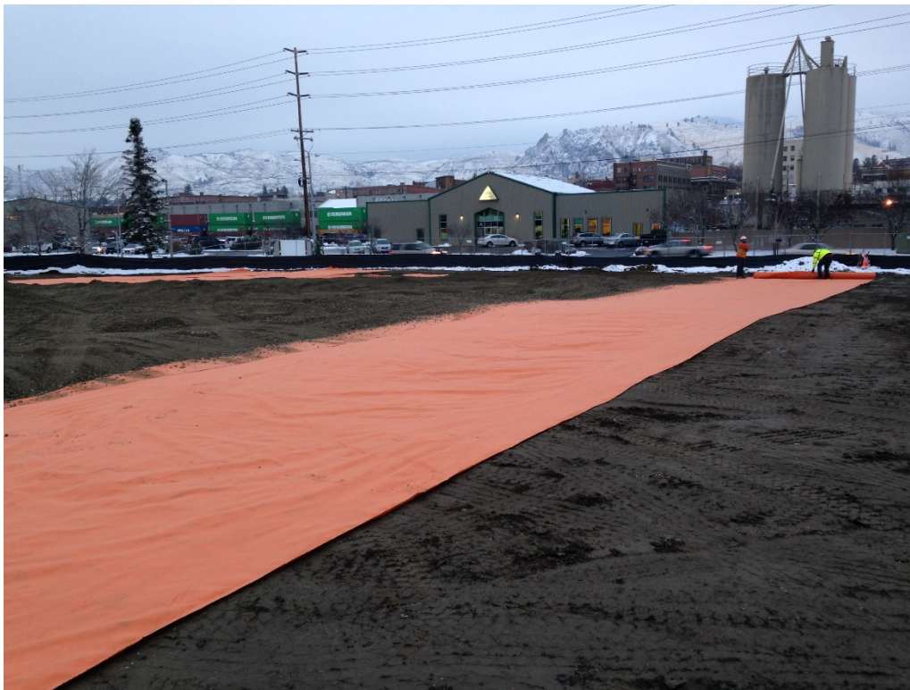
Figure 4: Demarcation Fabric Placement (12/02/2015)
