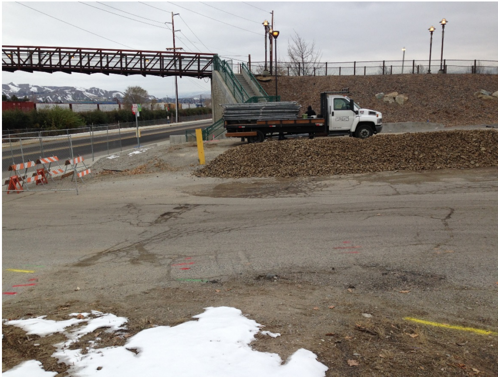
Figure 1: Construction Entrance Installation (12/01/2015)
