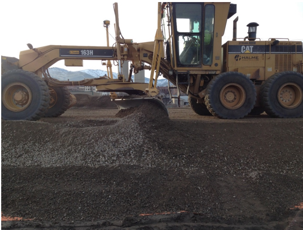
Figure 8: Cap Construction (12/15/2015)
