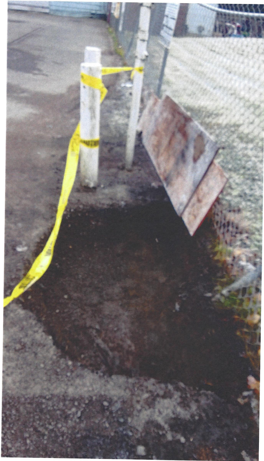
Picture 2. Excavation performed by Harrison Distributing.
