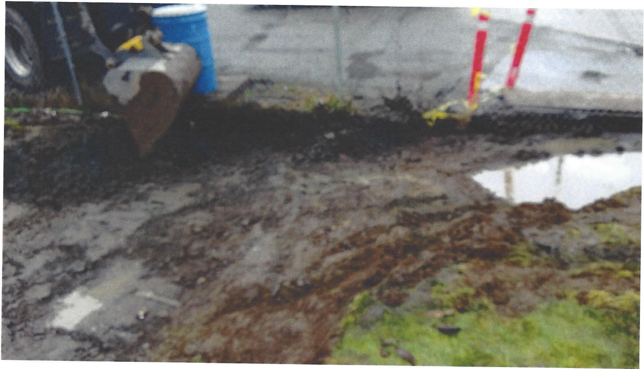
Picture 7. Excavation of non-paved contaminated area.
