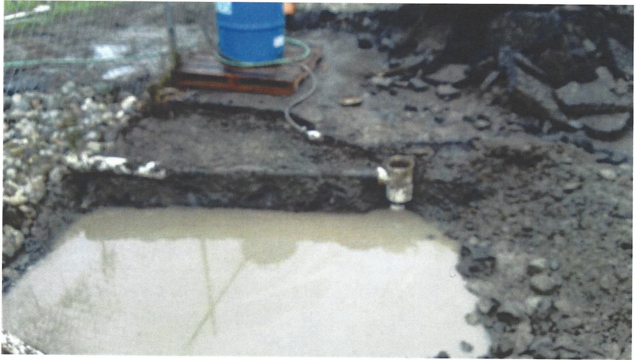
Picture 10. Excavation of paved contaminated area.
