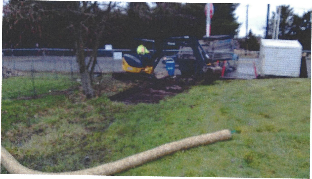
Picture 6. Excavation of downstream surface water swale.
