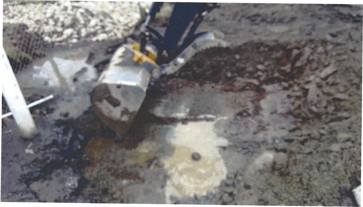
Picture 8. Excavation of paved contaminated area.
