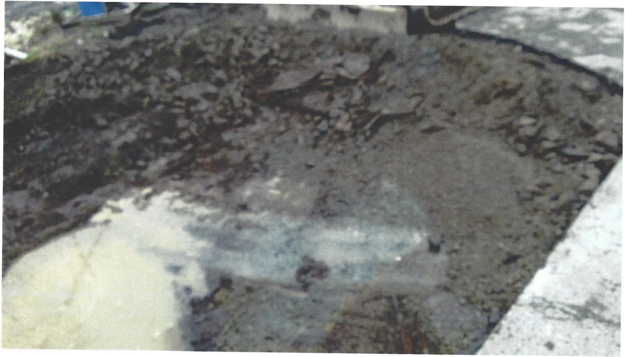
Picture 9. Excavation of paved contaminated area.
