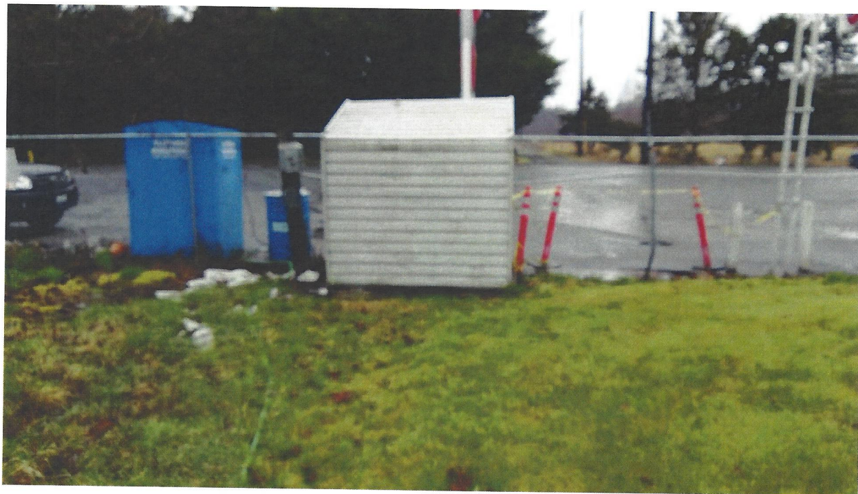
Picture 5. Downstream surface water discharge swale before excavation. Diapers placed in swale to absorb surface contamination.
