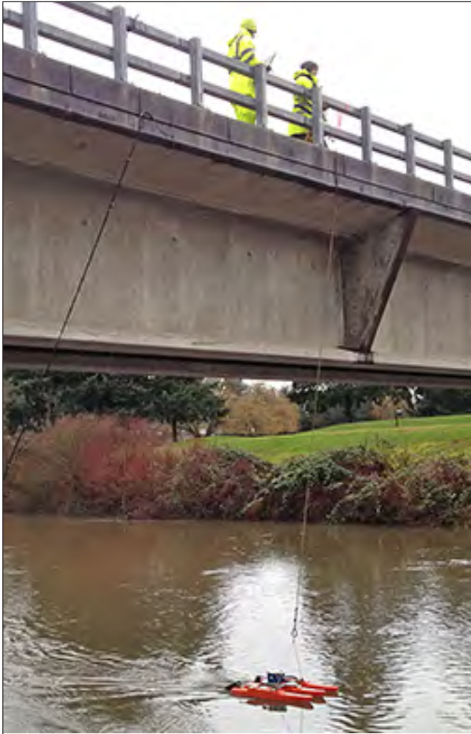
Figure 2. U.S. Geological Survey field personnel measuring streamflow at the Duwamish River at Golf Course at Tukwila, Washington (12113390), at river kilometer 16.7. Photograph by Kathleen Conn, U.S. Geological Survey, January 11, 2014.
