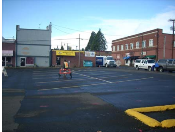
Photo #1: View of the northwestern area of the Pick-Rite Thriftway property – former Flying A gas station area. Geophysicist conducting an electromagnetic survey to identify locales of potential abandoned fuel tank.
