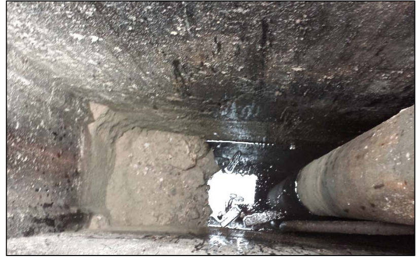
10. Concrete vault of former hydraulic hoist in central portion of subject property
