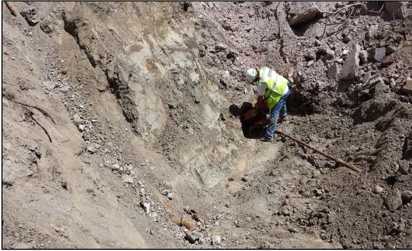
13. Former UST3 location in northeast portion of the subject property – Looking South
