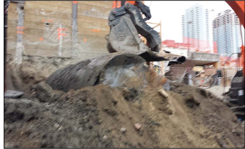
6. UST2 was removed from the subject property - Looking West
