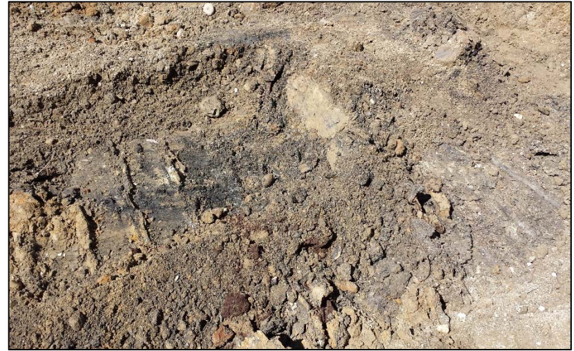
2. Contaminated fill soil in north portion of mass excavation - Looking West
