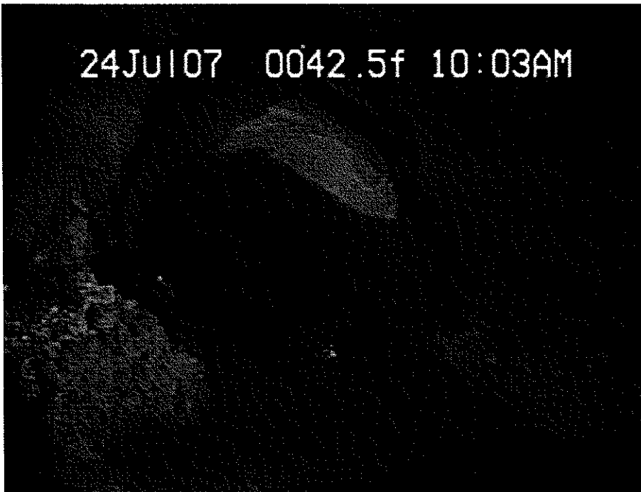
Photograph E-08: Lateral line section from DSI-19 to the main-line at catch basin DSI-21. This lateral line is approximately 12-inch diameter concrete-reinforced wood pipe.
