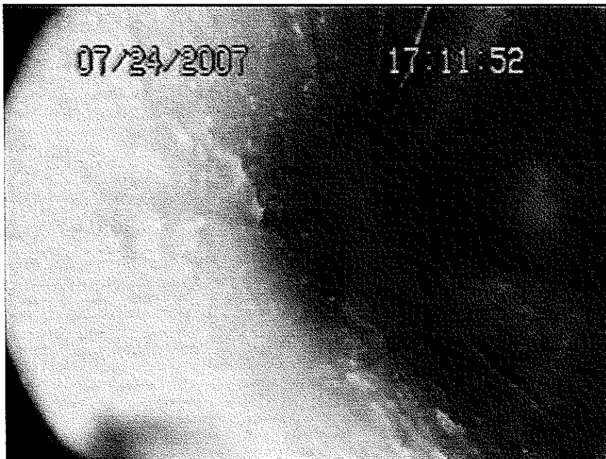
Photograph E-08: Lateral line section from DSI-19 to the main-line at catch basin DSI-21. This lateral line is approximately 12-inch diameter concrete-reinforced wood pipe.
