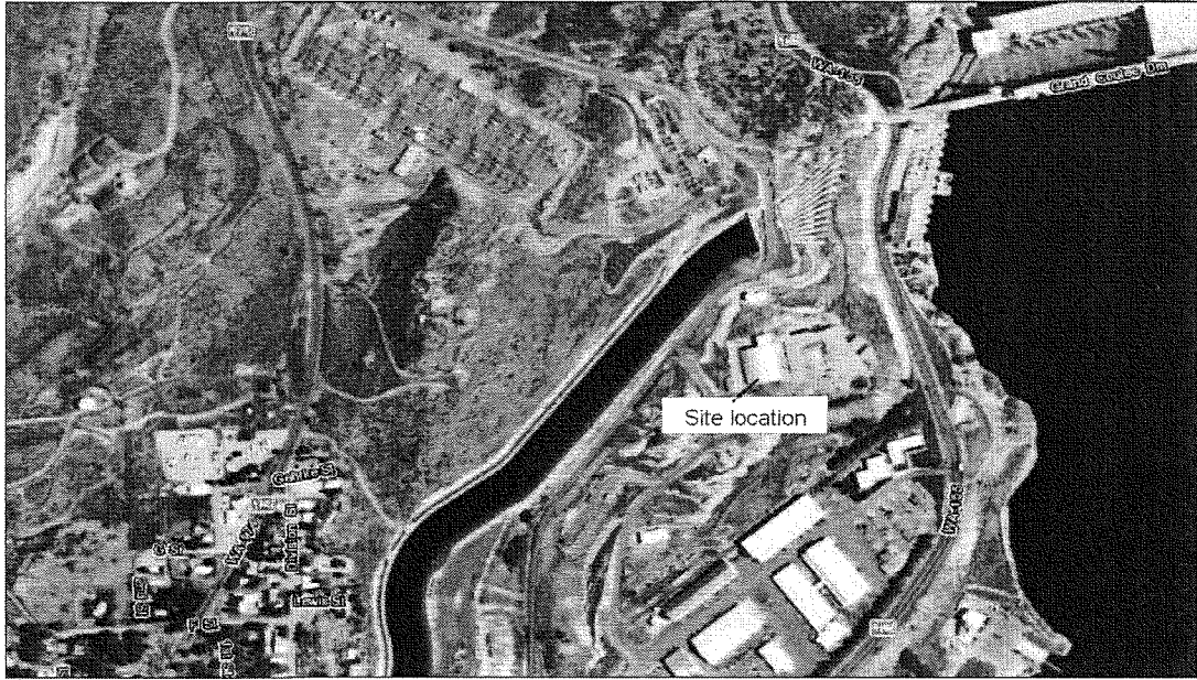
BPA Maintenance Facility
