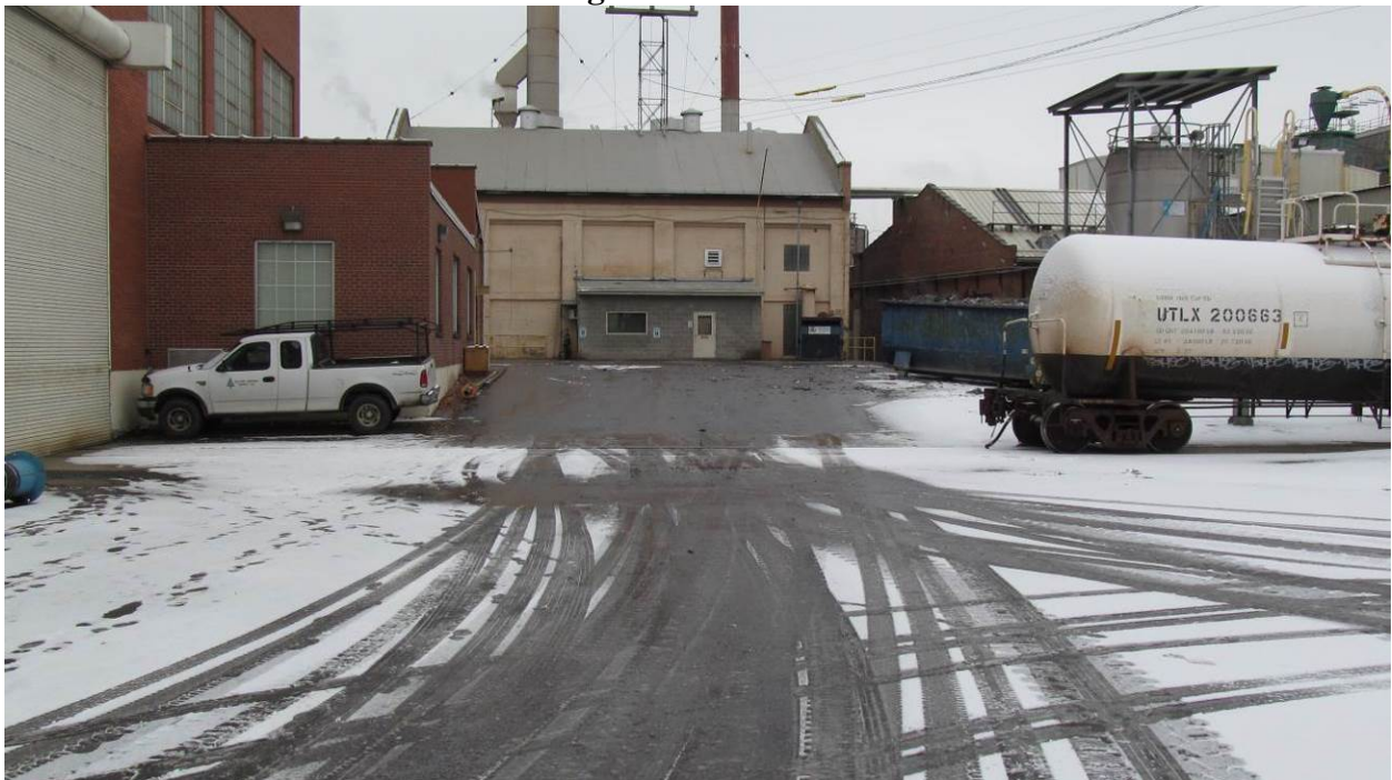
Photo 4: Boiler Room and Surrounding Area – from the south
