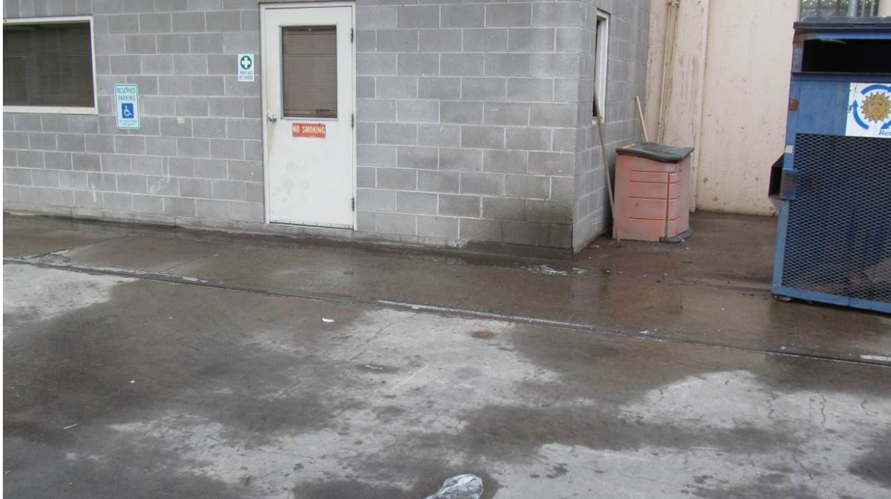
Photo 1: Boiler Room East Side - from the southeast
