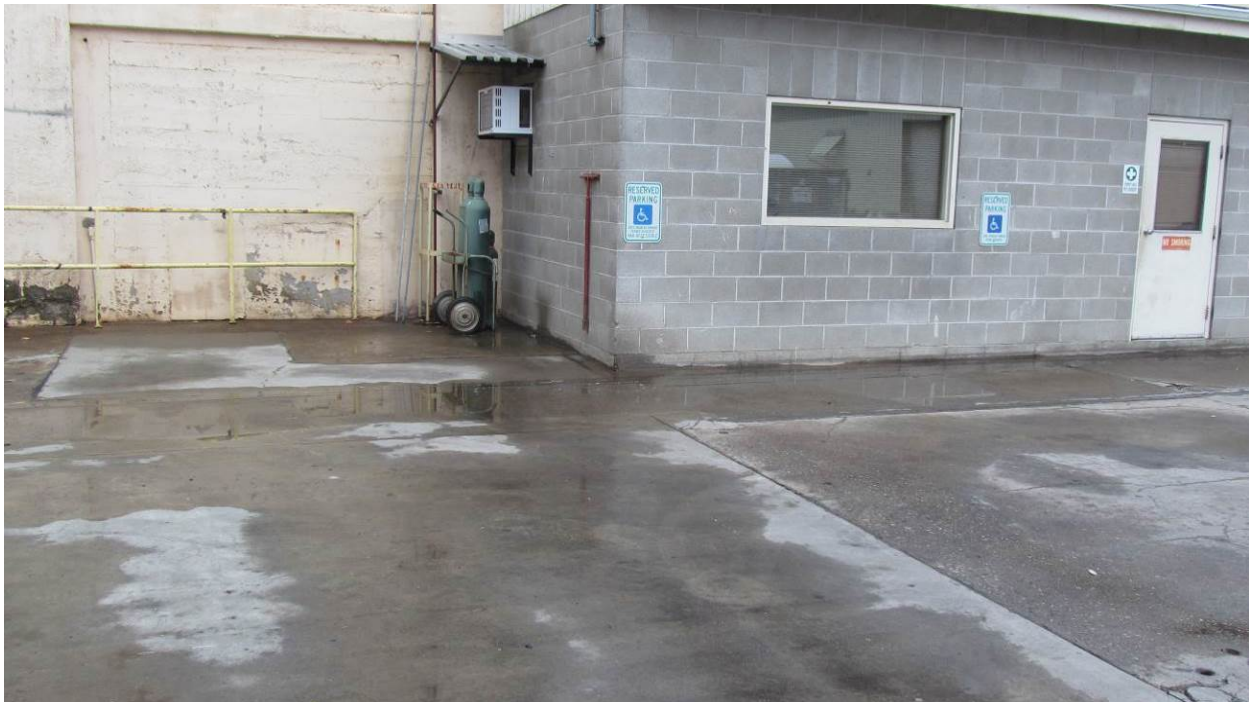
Photo 2: Boiler Room West Side - from the southwest
