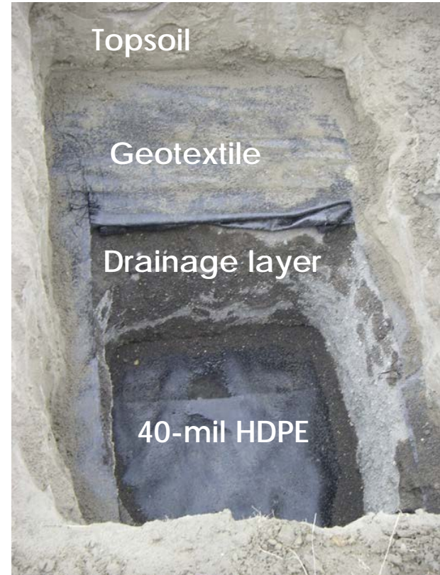
Zone A Cover System Test Pit
