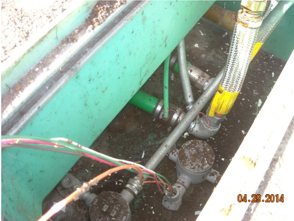
Photo 11 View of dispenser island sump.
