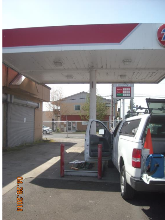
Photo 7 Looking west at the removed dispensers and canopy.
