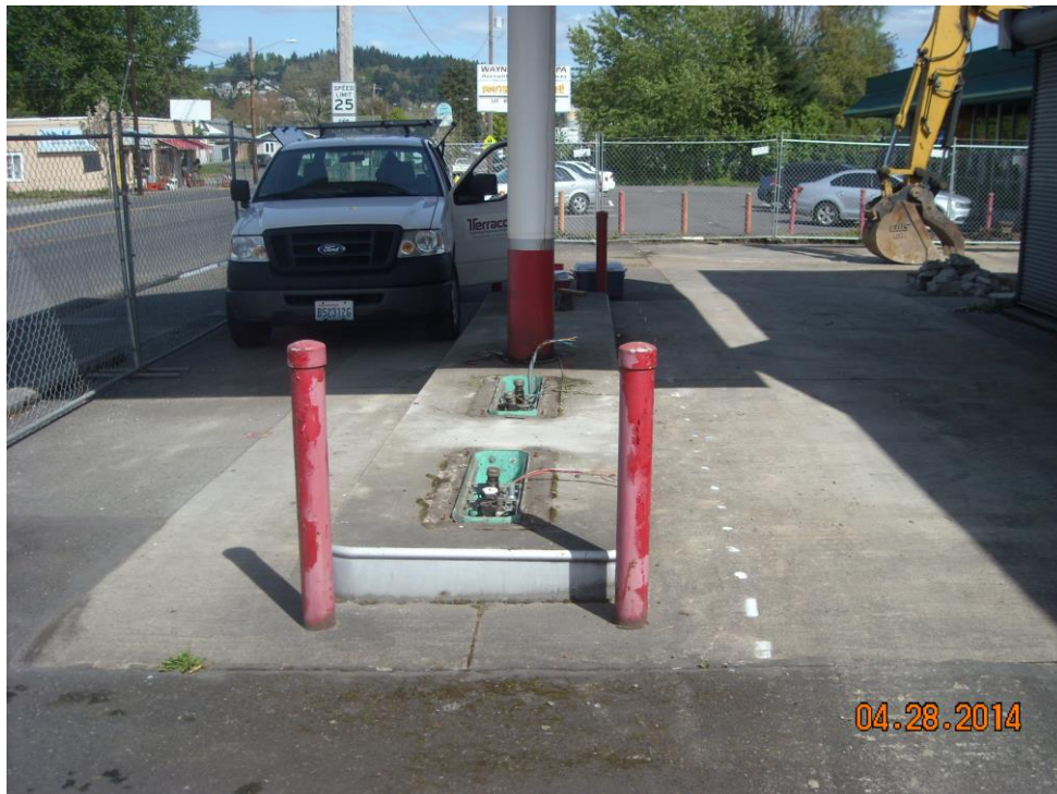
Photo 8 Looking east at the removed dispensers, UST complex in right background.
