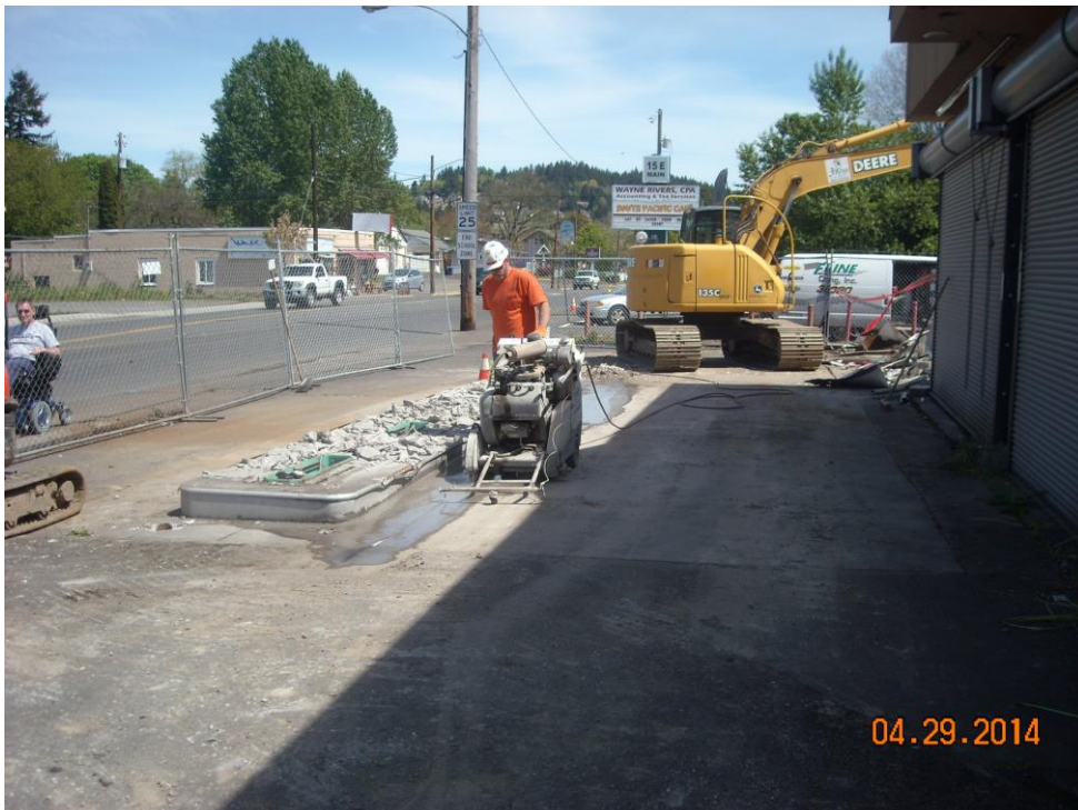
Photo 12 Looking northeast at dispenser island, breaking up/cutting concrete.
