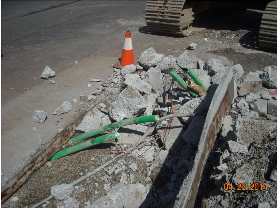
Photo 13 Looking northeast, pea gravel and green product piping exposed at dispenser island.
