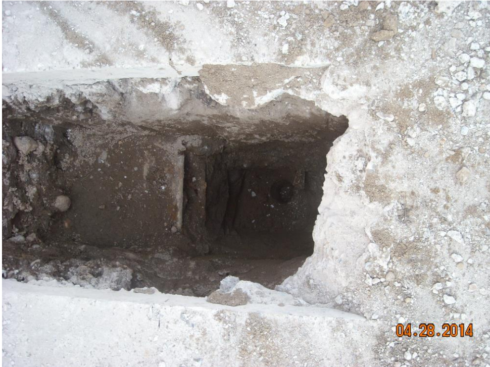
Photo 3 Looking into THW-5 sample location with groundwater in bottom.
