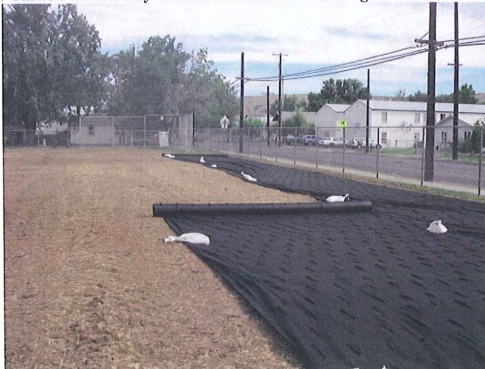
Photo D-2: Garfield Elementary School installation of marker geotextile.
