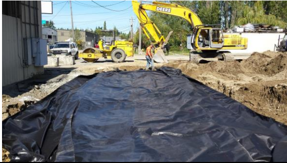
Photo #19: Three sheets of geotextile fabric running north south
