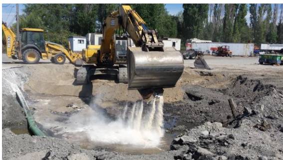
Photo #5: Mixing in ORC-Advanced to soil/groundwater
