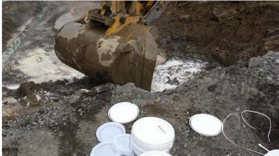
Photo #9: Mixing in ORC-Adv Pellets and RegenOx Part A and Part B.
