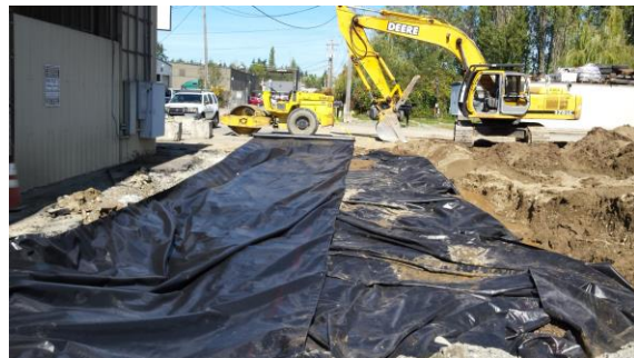
Photo #18: Fully wrapped soil/mulch mix with geotextile fabric running north south for bridging affect, stability.
