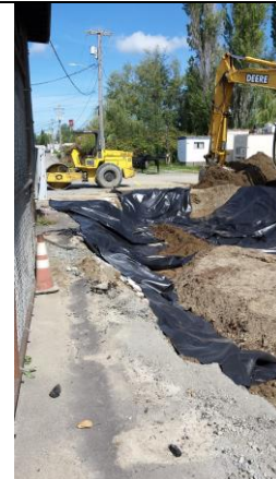
Photo #14: First placement of Soil/Mulch Mix extended to approx. 7-8 in excavation next to pipe. Below water table in picture.
