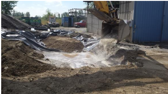
Photo #15: Mixing Regenesis chemicals in northern portion of excavation. 60% of total chemicals placed here due to previous analyticals being well above MTCA lean up levels.
