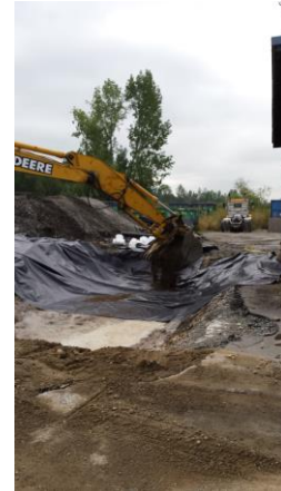
Photo #14: First placement of Soil/Mulch Mix extended to approx. 7-8 in excavation next to pipe. Below water table in picture.
