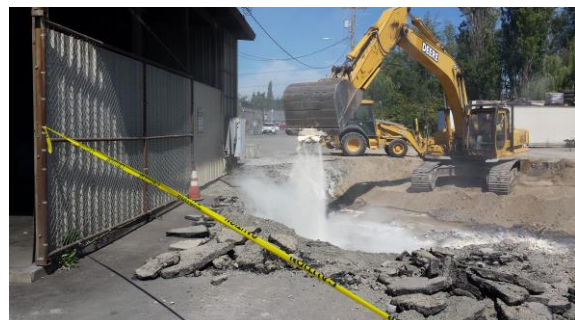
Photo #6: Mixing In ORC-Advanced to north
