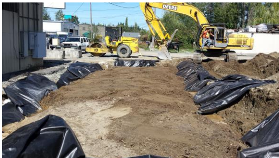
Photo #17: Filled to 2 feet below finish grade for structural fill placement.
