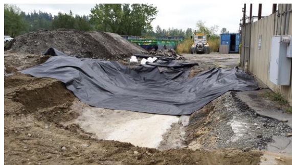
Photo #12: Laying base of Permeable Membrane Filter PMF
