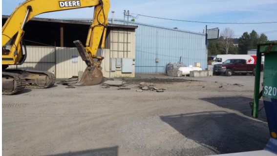
Photo #1: Removing asphalt (uncovering AEG MW-3)
