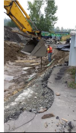
Photo #8: Resetting stormwater pipe grade
