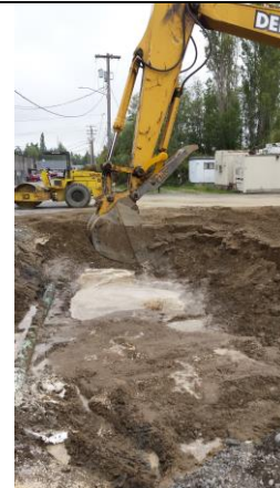
Photo #10: Frothing of groundwater creating a brown color, many bubbles forming.
