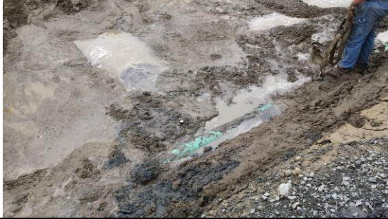
Photo #7: After ORC-Adv. Mixed in east of stormwater pipe (green) note oil residue seeping from west of pipe creating sheen near pipe.
