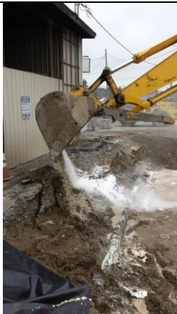
Photo #11: Sidewall distribution of ORC-Advanced and RegenOx products
