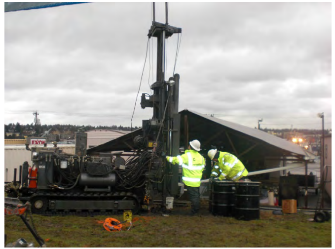
Photograph 8. Drilling south of Former Barreling Shed #3 viewing north
