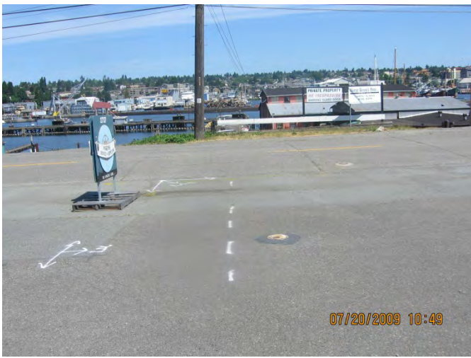
Photograph 1. North portion of ASKO Hydraulic Property and the West Commodore Way ROW viewing north.
