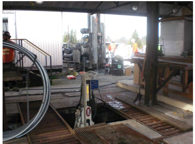
Photograph 4. Advancing borings on the interior of Former Barreling Shed #3 viewing west.
