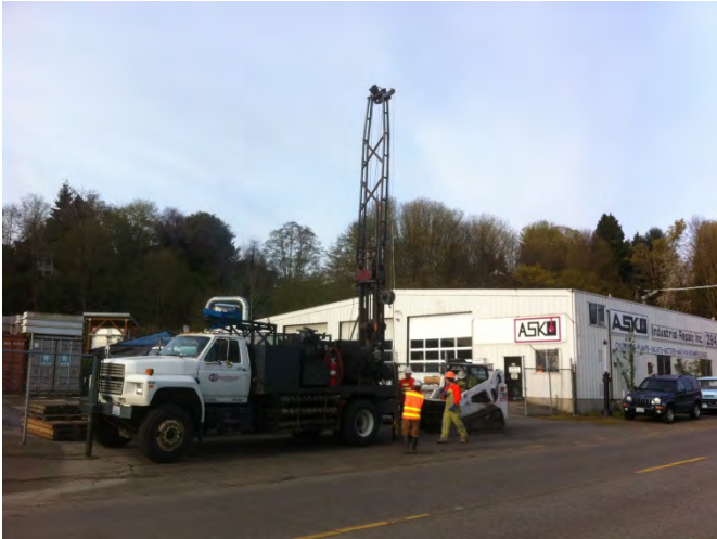
Photograph 9. Drilling in the vicinity of ASKO Industrial Repair viewing southwest.
