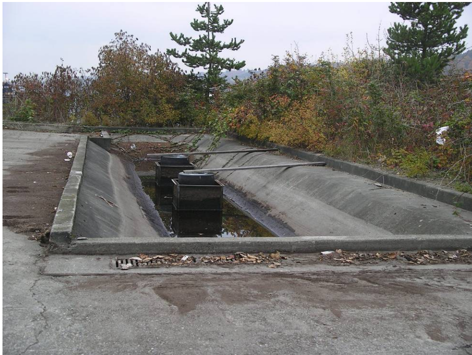
Photo 4: Stormwater Collection Basin – from the southeast
