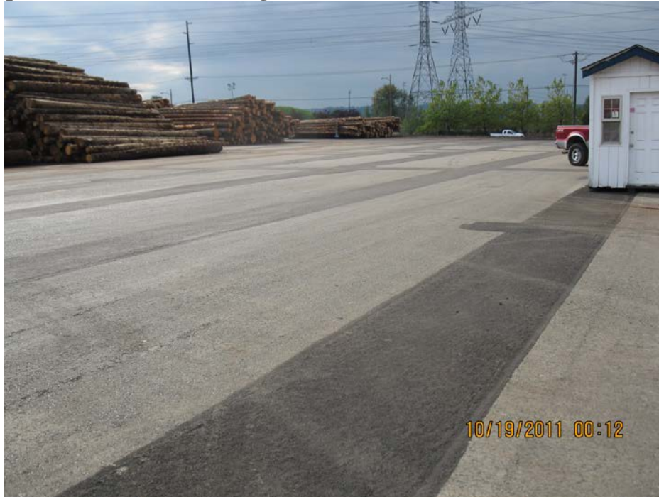
Photo 1: Cap Area and Lumber Storage Area - from the northeast
