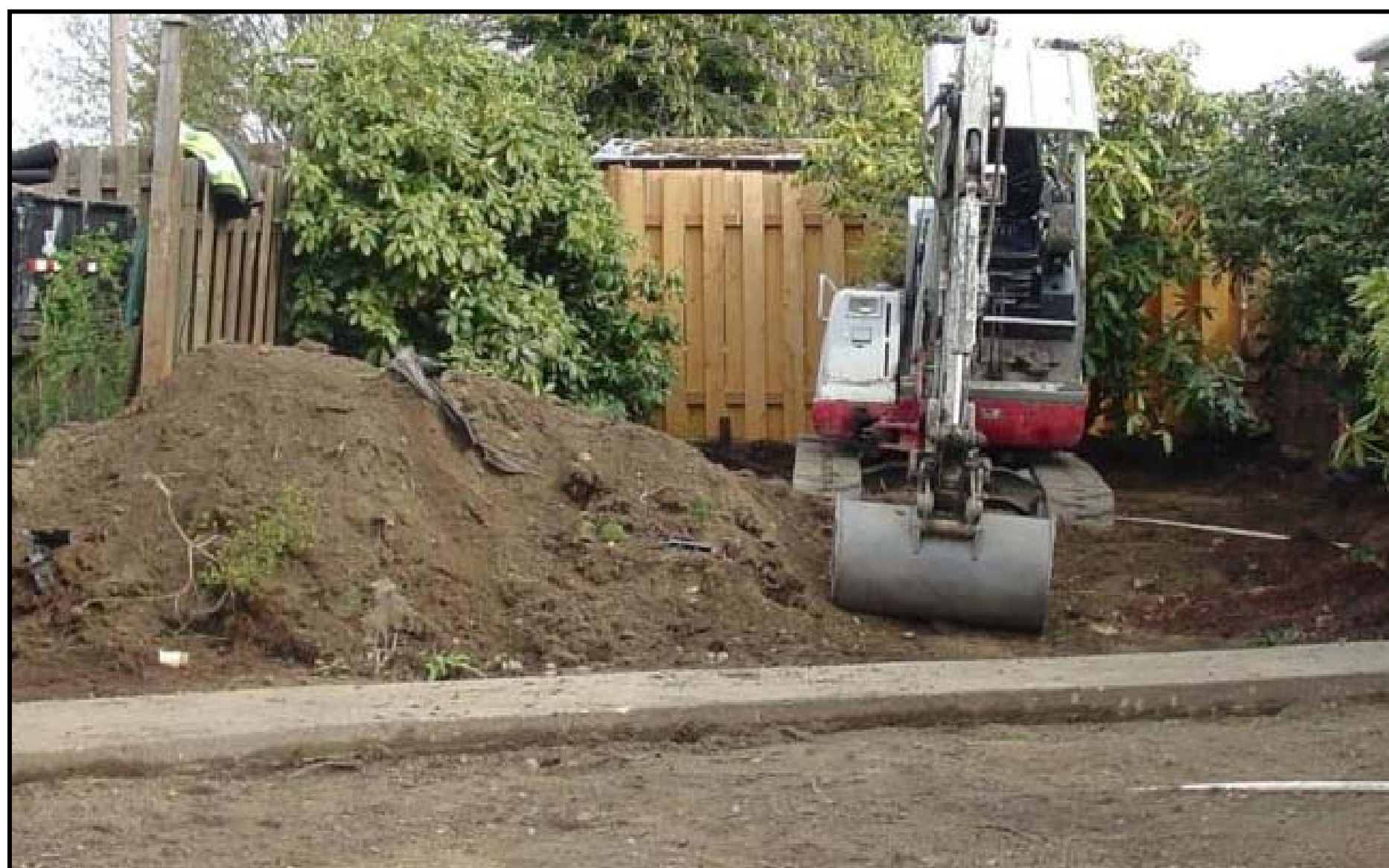
Ecology's contractor digs out contaminated soil, which goes to a landfill.
