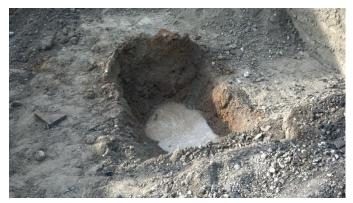
350 gallon UST excavation, water from tank cleaning
