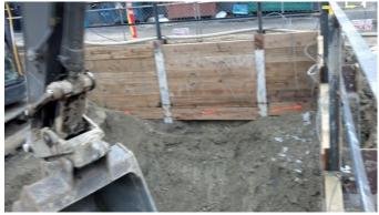
Subsequent UST soil excavation area after shoring installation
