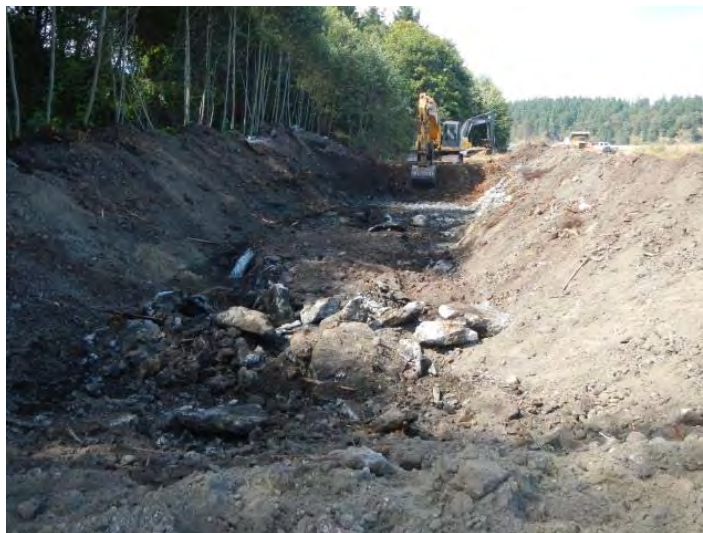
Infiltration ditch
