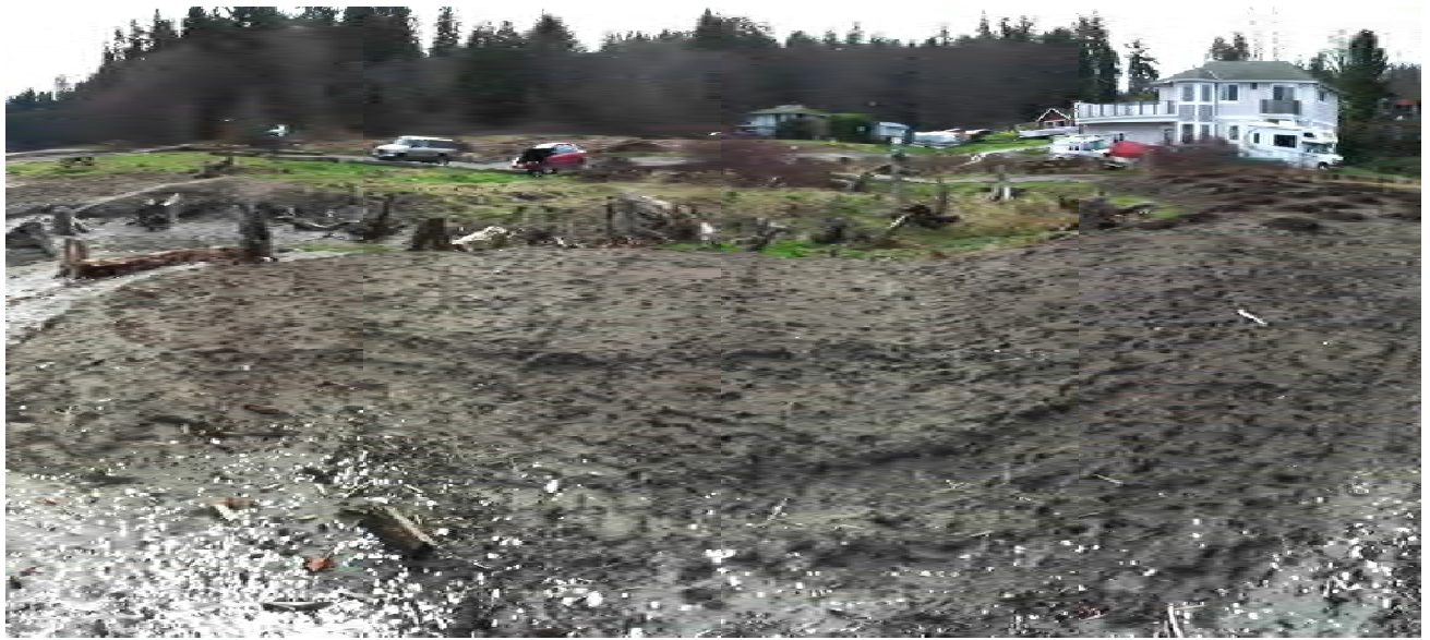
Photograph 9 Restored portion of the northern drainage swale viewed from the north.
