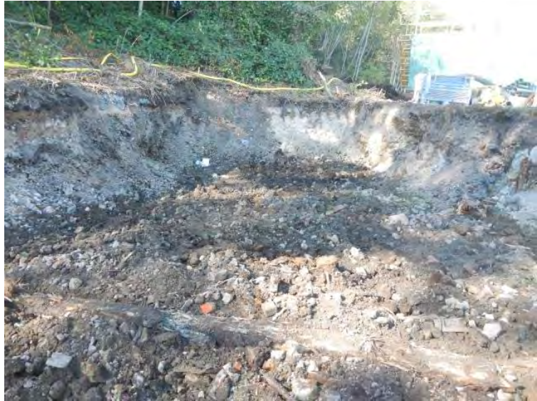
Northwest extent of Metals Area excavation (see Figure 7)
