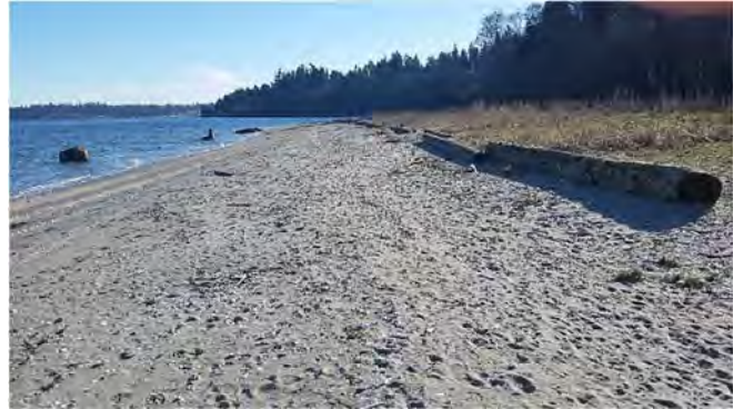
Shoreline after grading activities
