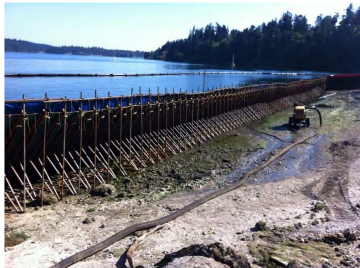
Portadam installed to complete nearshore sediment excavation
