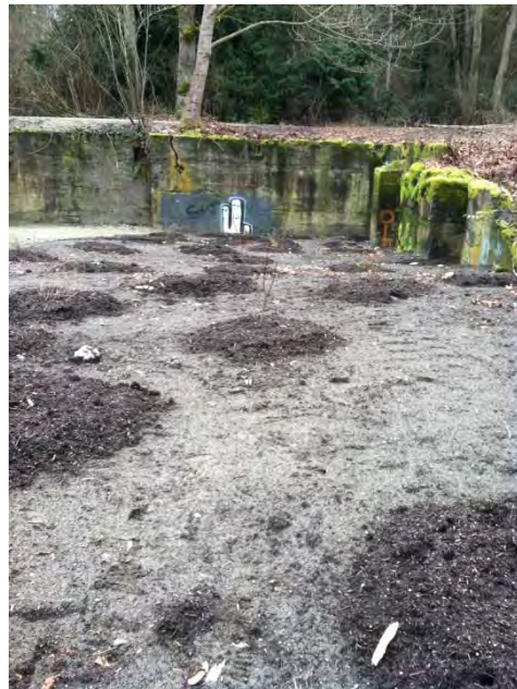
Photograph 15 Monitoring station 1 looking southeast.
