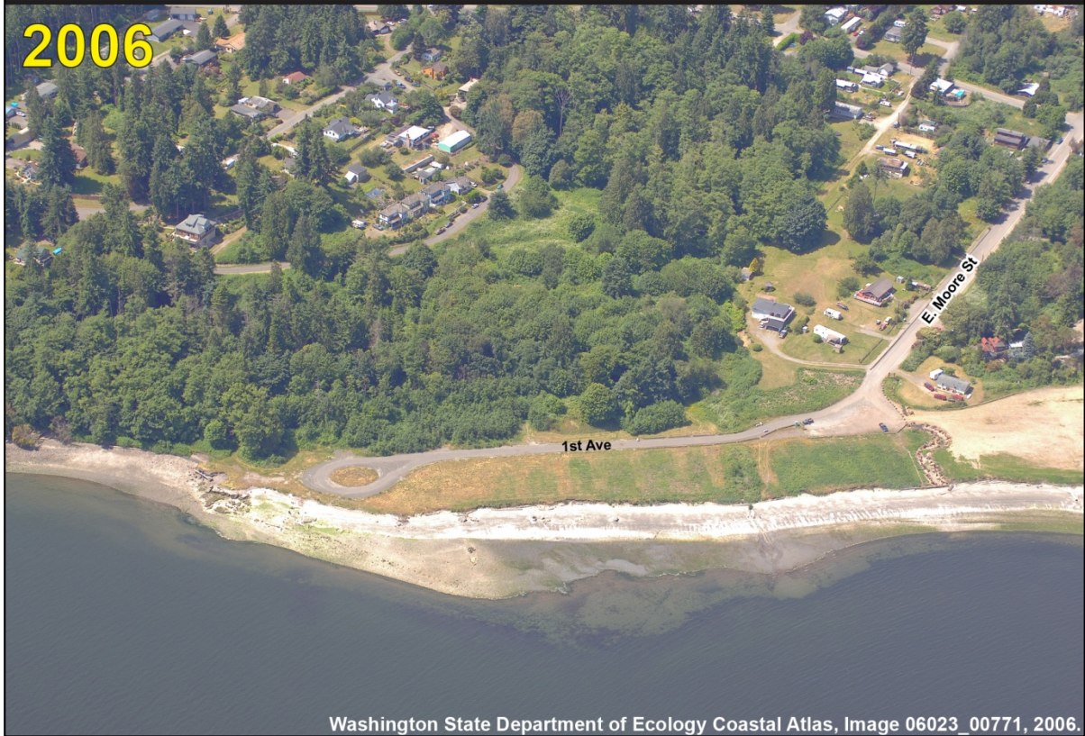
Figure 11. WDFW restoration project north of Irondale, in 2001 before restoration work, and in 2006 after restoration work.
