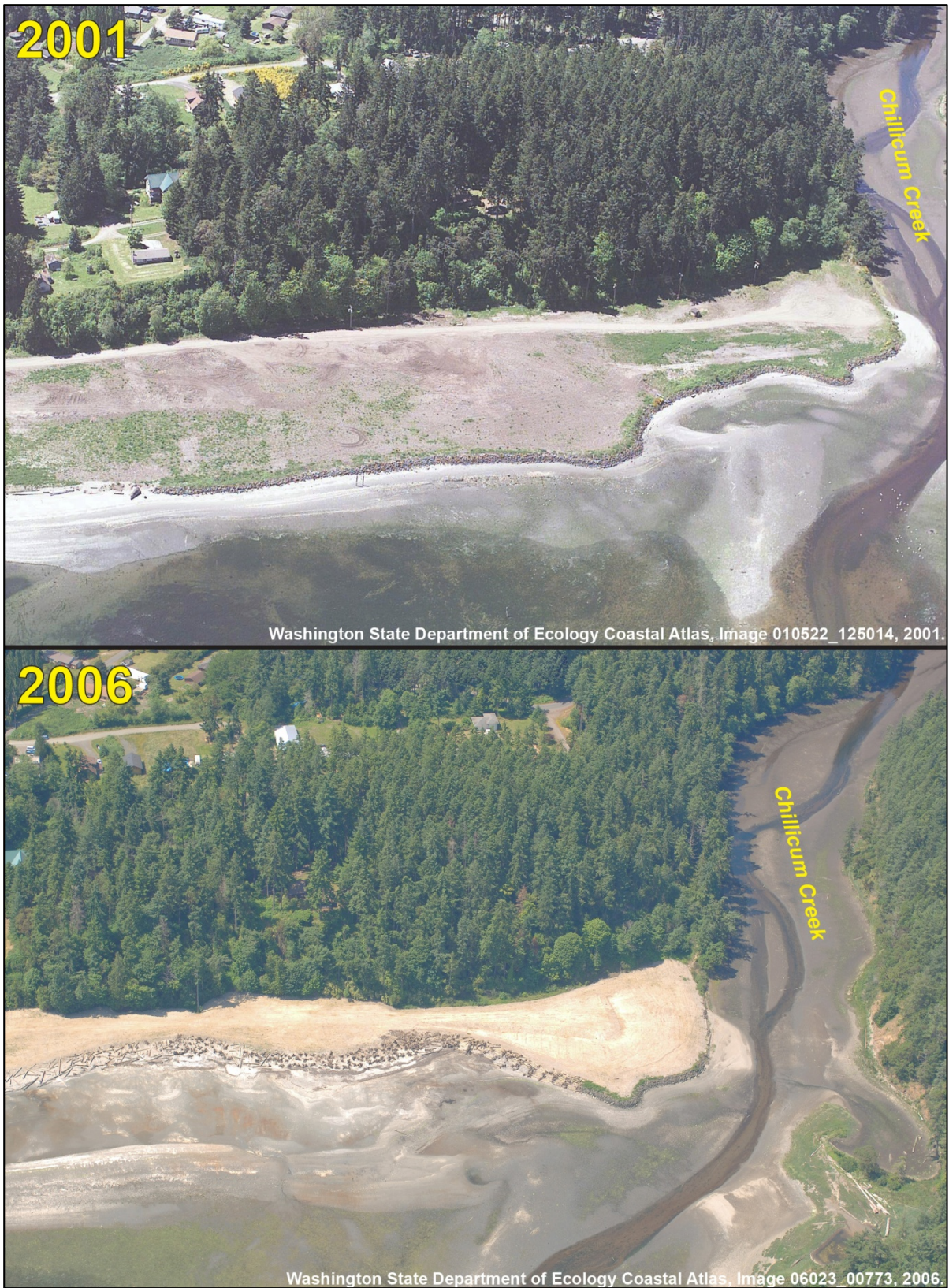
Figure 13. WDFW restoration project north of Irondale, in 2001 before restoration work, and in 2006 after restoration work.
