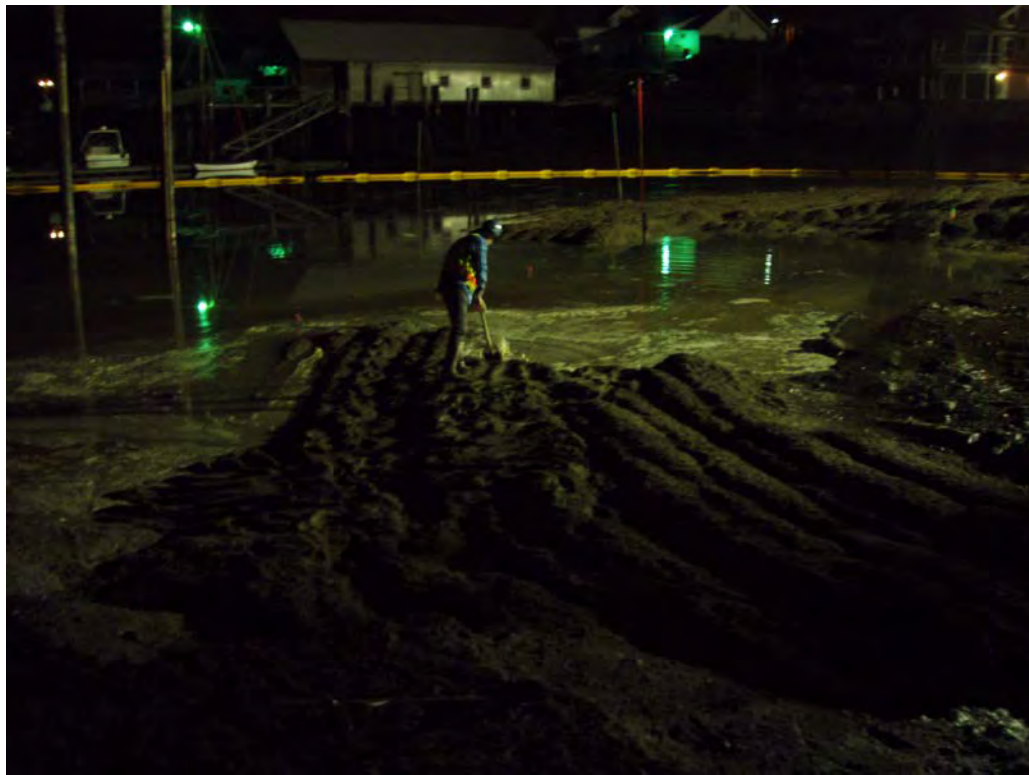
October 17, 2008. Placement of the sand cap.
