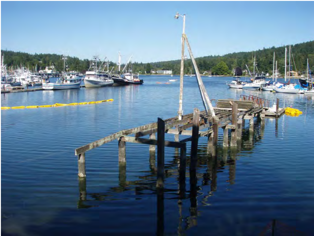
September 15, 2008. Pier awaiting arrival of crane and marine demo crew.
