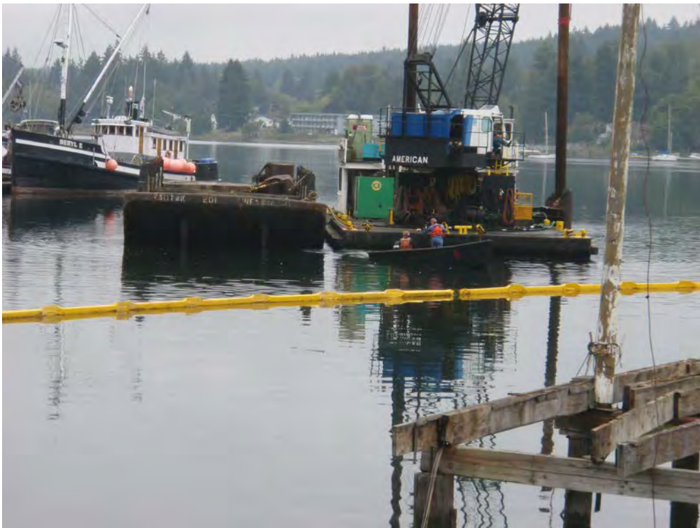
September 22, 2008. Arrival of the crane and barge for demo and dredging.
