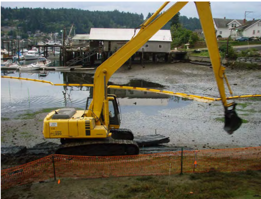
September 24, 2008. Excavation of sediment near the marsh and wetland.
