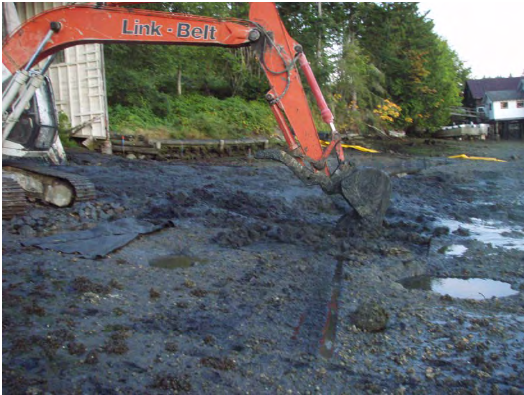
September 24, 2008. Removal of small railway piles.
