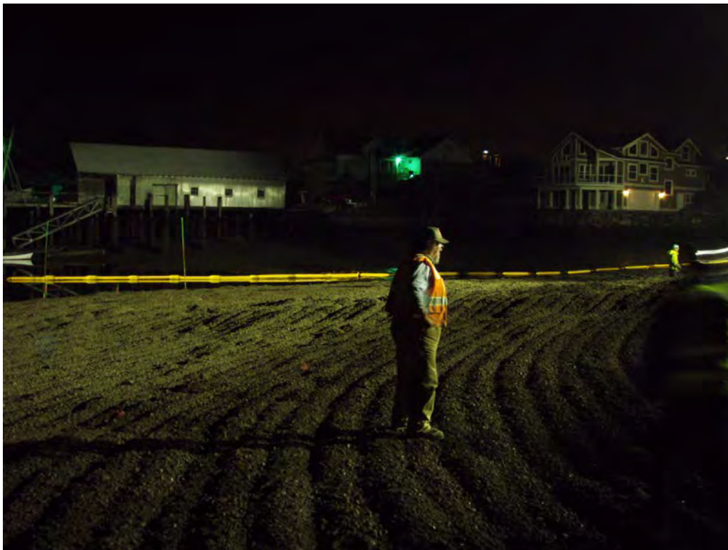
October 18, 2008. Cap after the rock mix was placed.
