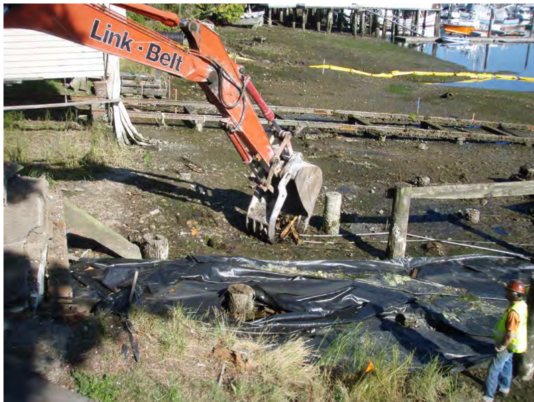
September 15, 2008. Removal of the small railway piles from land.
