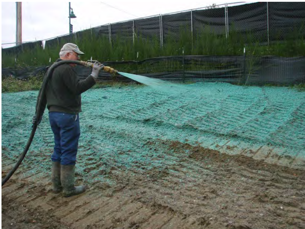
November 6, 2008. Application of the hydroseed after completion of soil disturbing activities.
