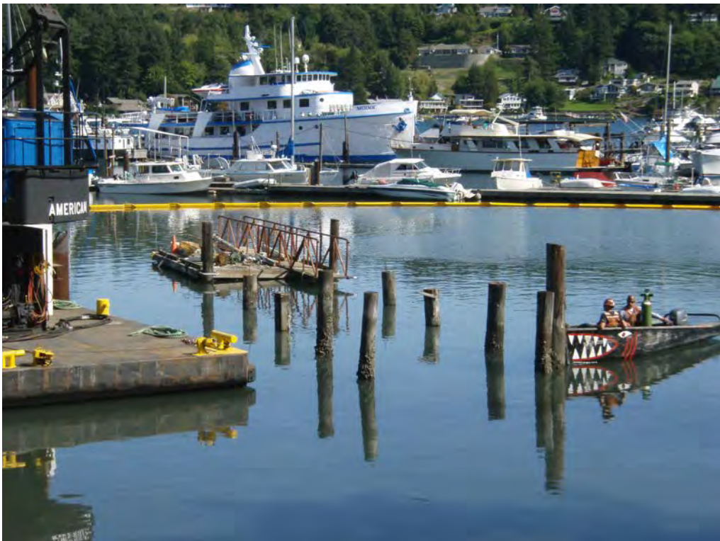
September 22, 2008. Removal of pier piles.
