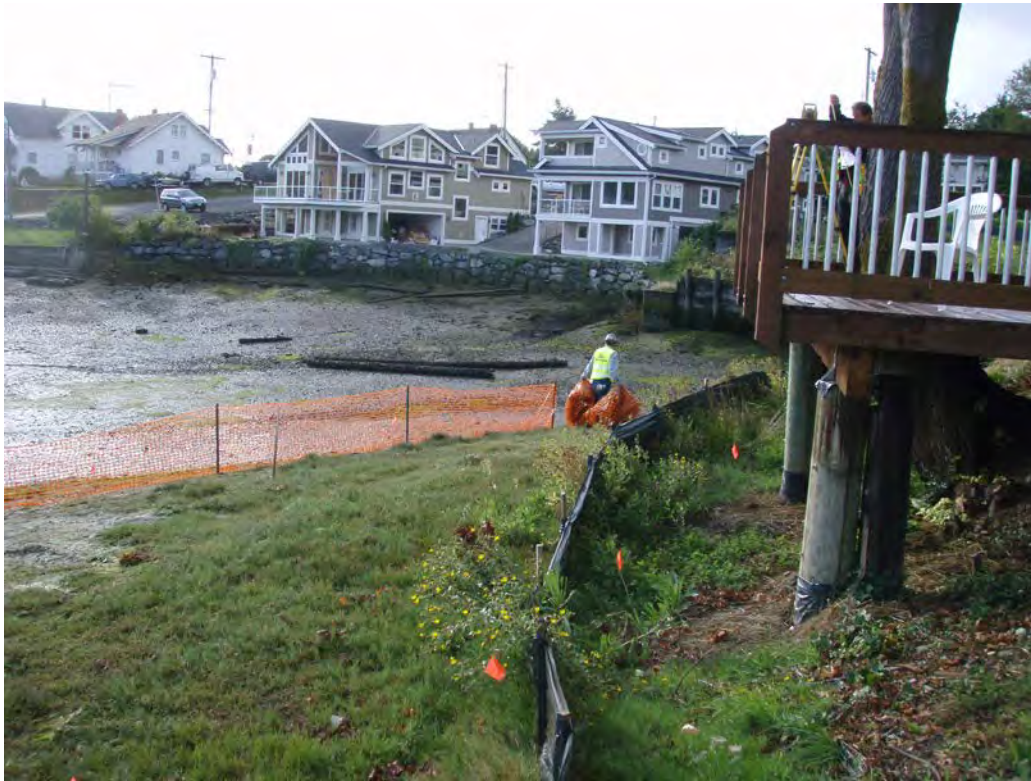
September 5, 2008. Installing Hig-vis-fence to protect the marsh and wetland.
