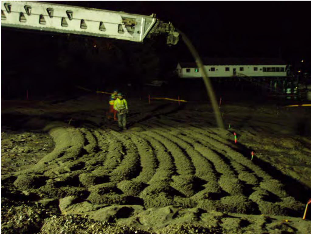
October 18, 2008. Placement of the sand cap.
