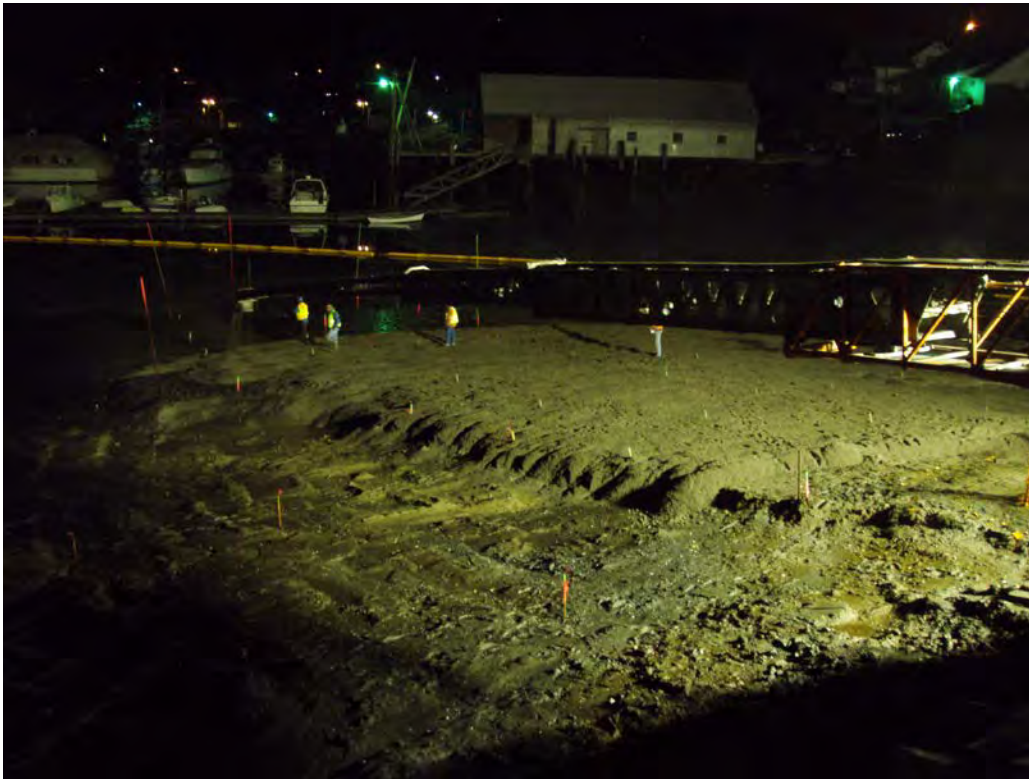
October 17, 2008. Placement of the cap using the telescoping conveyor belt.
