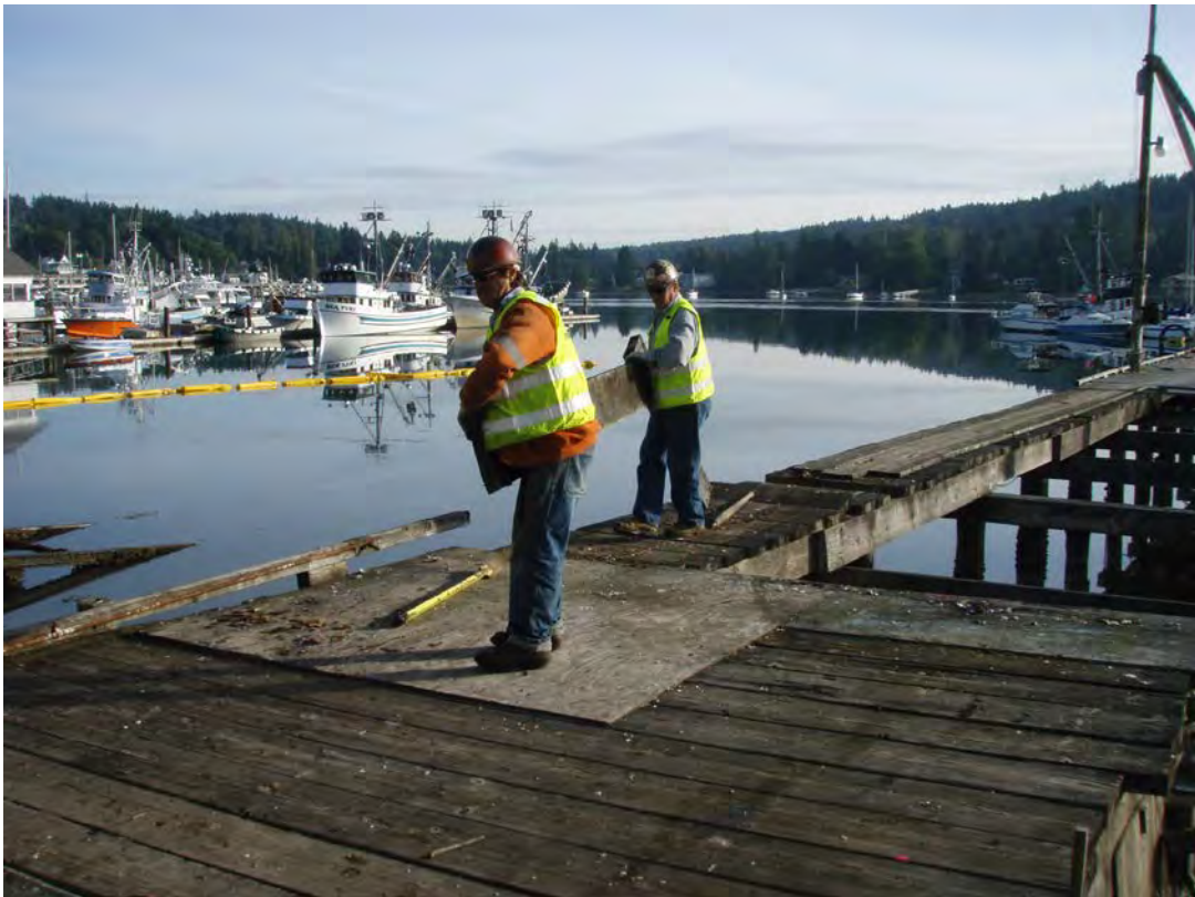
September 5, 2008. Demo of the pier decking.
