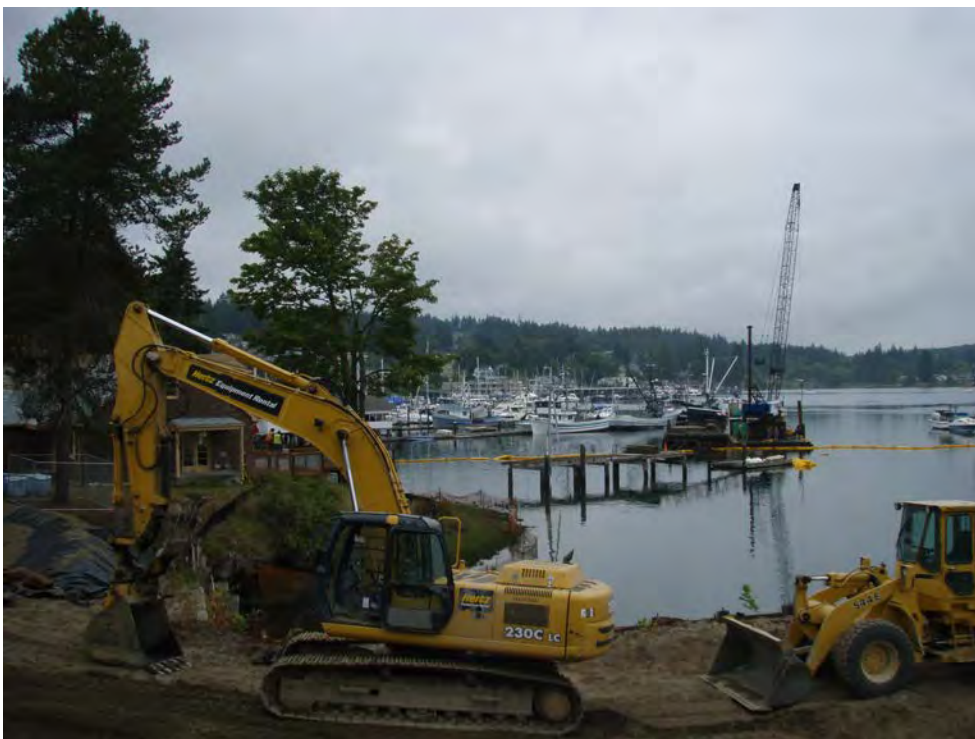
September 19, 2008. Upland excavation equipment staged for night capping work.
