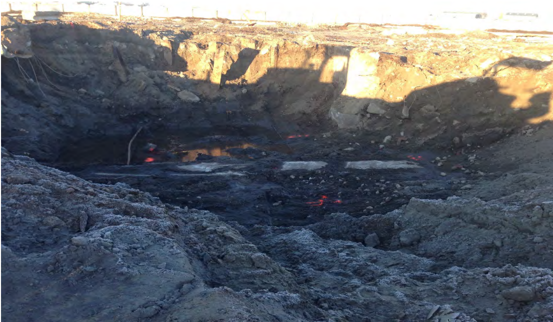
Photograph 28– UST 70 excavation: looking west
