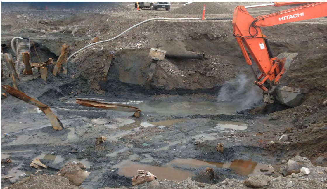
Photograph 26 – UST 29/Latex excavation: looking south
