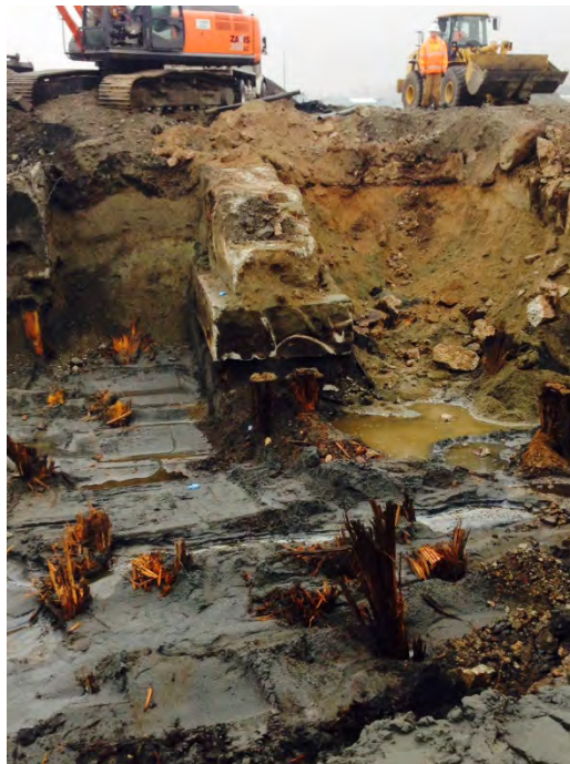
Photograph 32 – USTs 71, 72, 73 excavation: bunker-contaminated soil beneath one concrete monolith on northeast side
