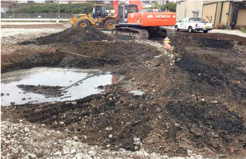
Photograph 21 – REC2-MW-5 excavation: looking east
