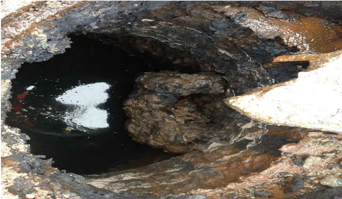
Photograph 13 – Hydraulic Barker Vault excavation: oil at vault location
