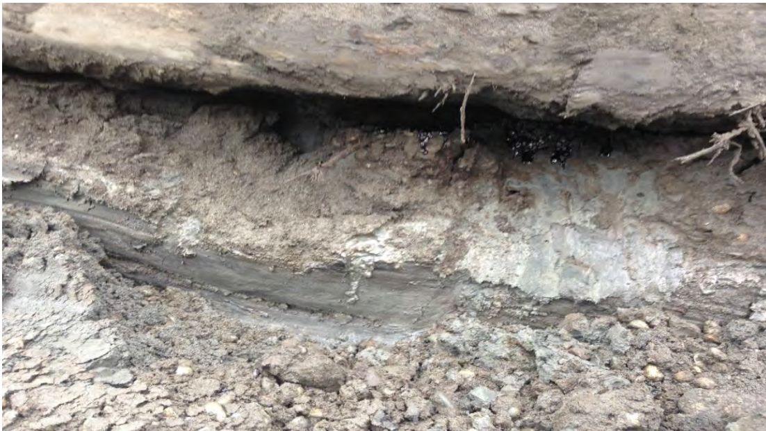
Photograph 31 – USTs 71, 72, 73 excavation: thin layer of bunker-contaminated soil under southern concrete monolith
