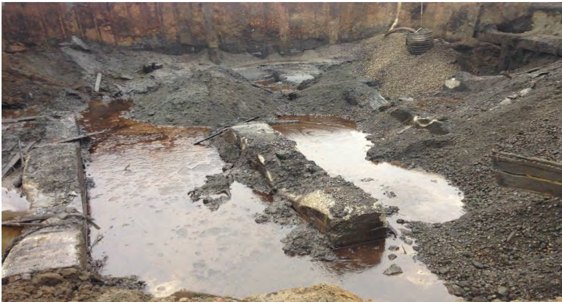
Photograph 30 – USTs 71, 72, 73 excavation: concrete tank saddles for former railroad car USTs
