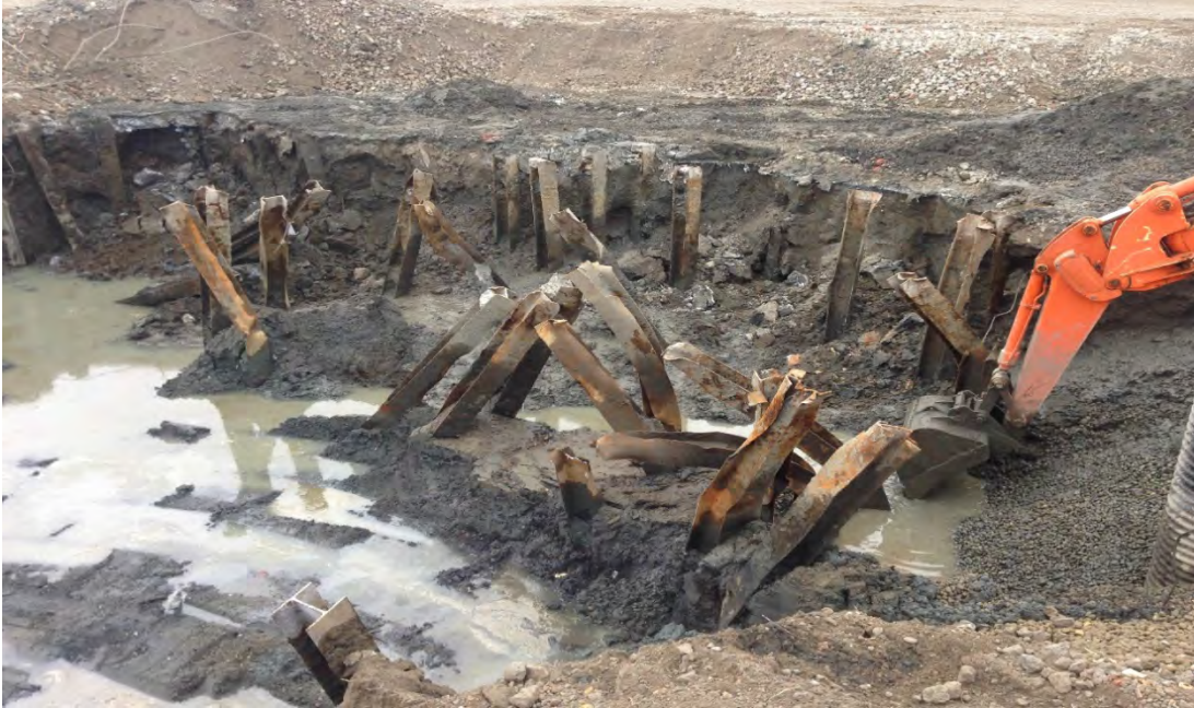
Photograph 23 – UST 29/Latex excavation: looking north
