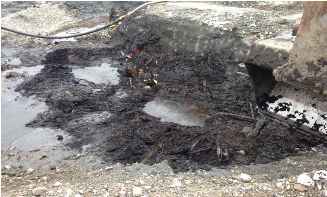
Photograph 10– CN-B2 excavation: concrete foundation monolith and lumber
