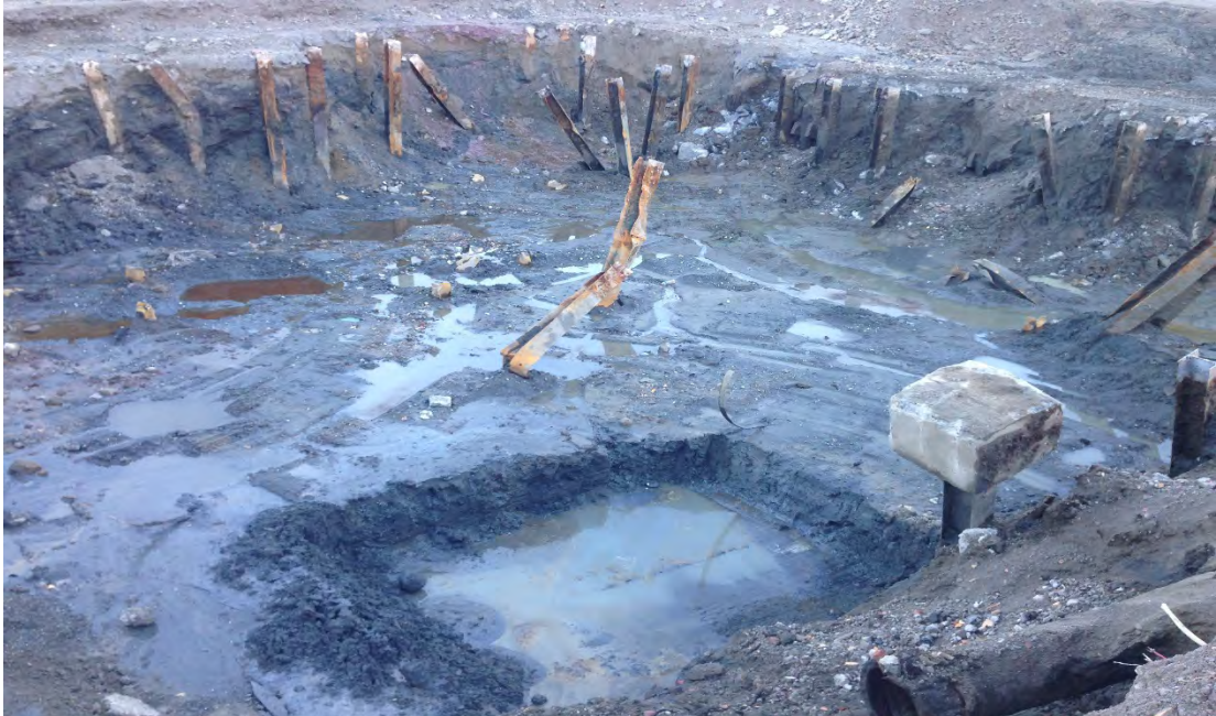
Photograph 25 – UST 29/Latex excavation: looking northeast
