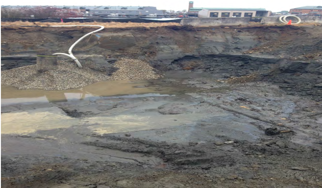
Photograph 16 – Naval Reserve South excavation: looking northwest
