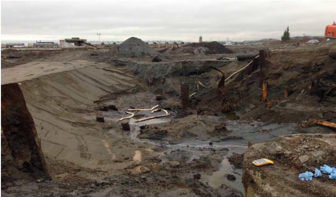
Photograph 33 – USTs 71, 72, 73 excavation: looking northwest (backfill on left)
