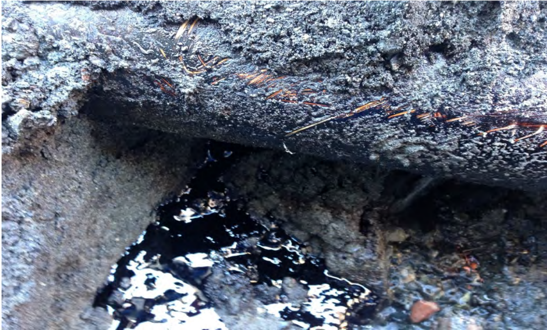
Photograph 5 – Bunker C ASTs excavation: bunker oil product
