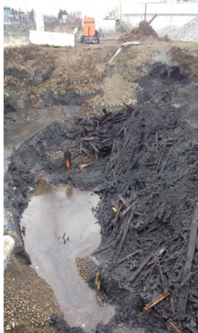
Photograph 15 - Naval Reserve Parcel UST excavation: lumber in eastern sidewall
