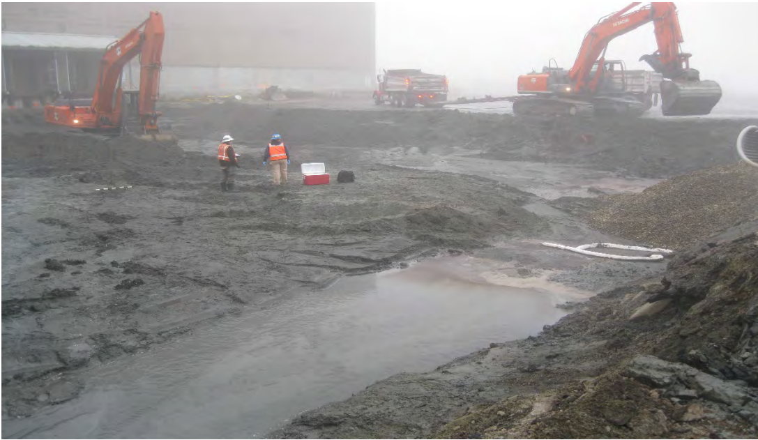
Photograph 7 – Bunker C ASTs excavation: east center of excavation looking southwest
