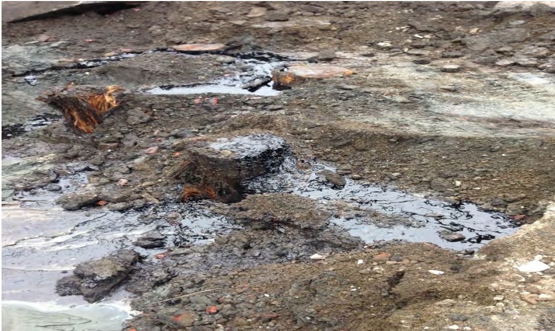
Photograph 6 – Bunker C ASTs excavation: pilings for former ASTs, with bunker oil
