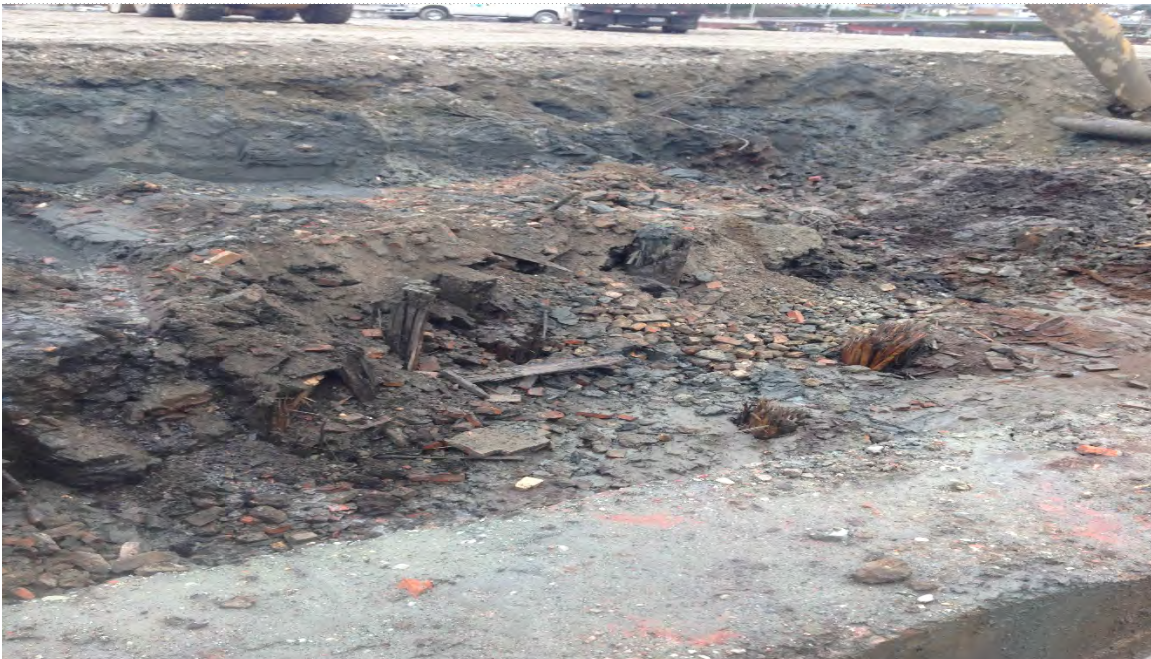
Photograph 8 – CN-B2 excavation: looking southeast
