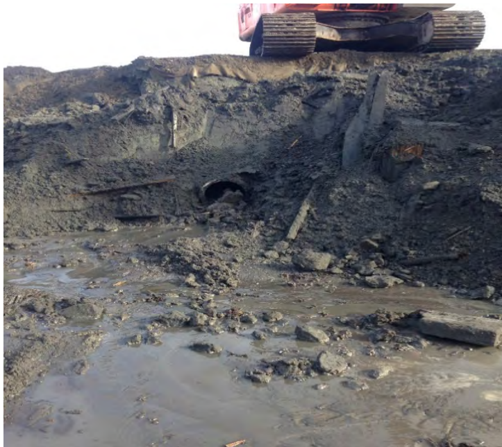
Photograph 24 – UST 29/Latex excavation: looking west
