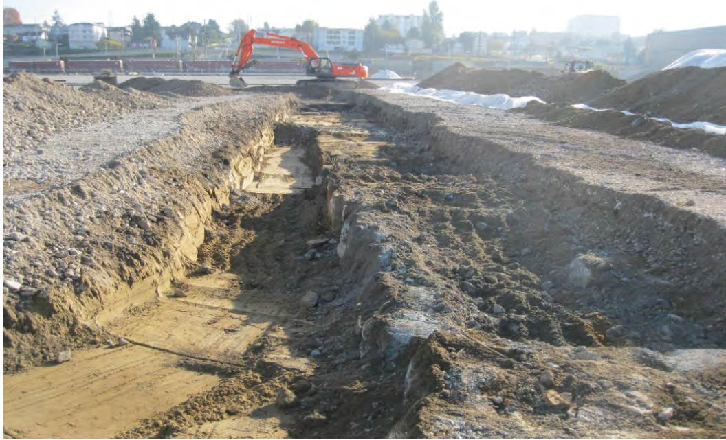
Photograph 3 – Boiler Baghouse Area excavation: looking east
