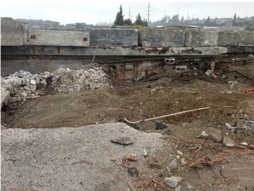
Photograph 20 – Rail Car Dumper excavation: looking north
