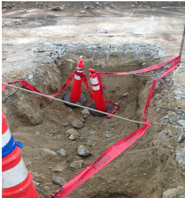
Photograph 12 – Heavy Duty Shop Sump excavation: looking north
