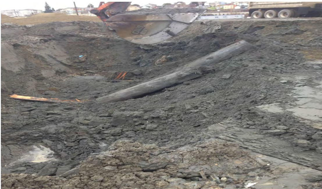
Photograph 18 – Naval Reserve South excavation: looking north
