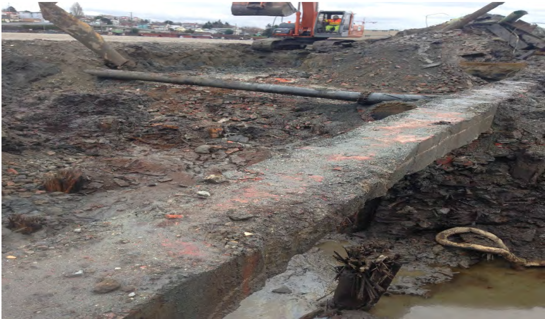
Photograph 9 – CN-B2 excavation: looking south
