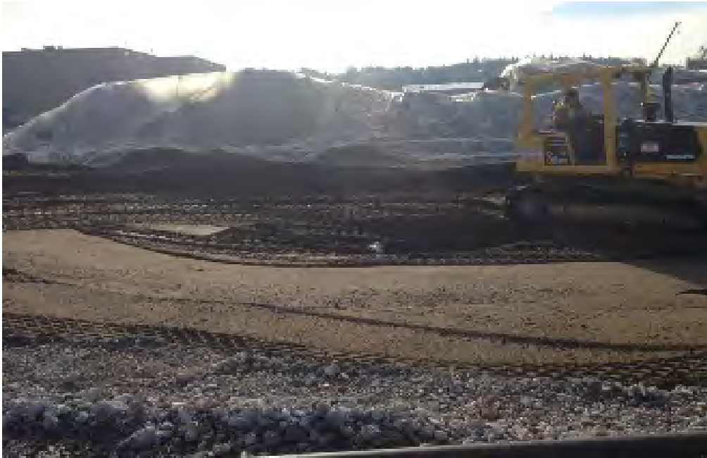
Photograph 1 – BA-MW6 Area excavation: backfilling
