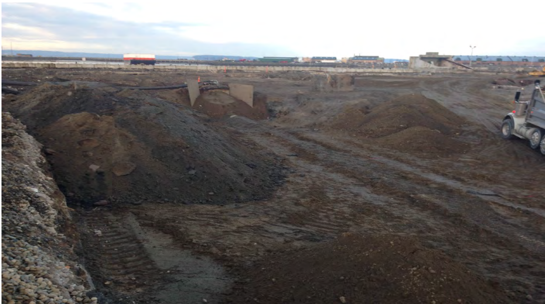
Photograph 34 – USTs 71, 72, 73 excavation: CSO pipe bypass and replacement
