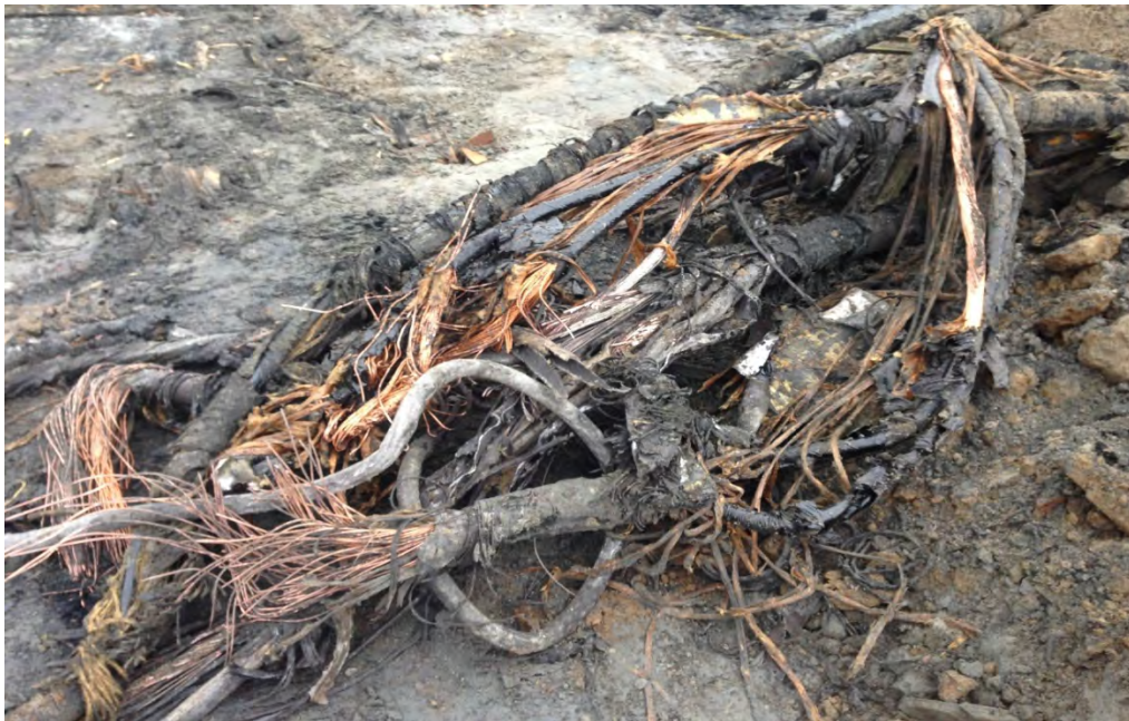
Photograph 4 – Boiler Baghouse Area excavation: copper wire in east end
