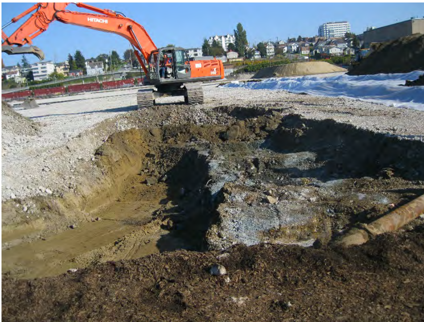
Photograph 2 – Boiler Baghouse Area excavation: looking east
