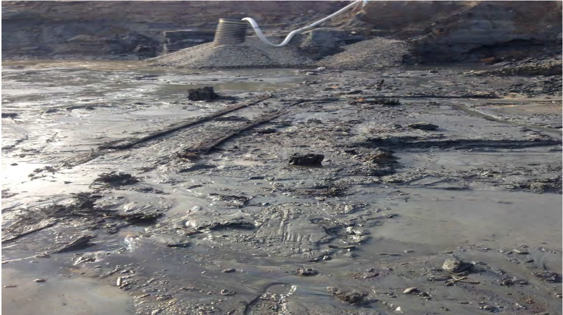
Photograph 17 – Naval Reserve South excavation: looking southwest
