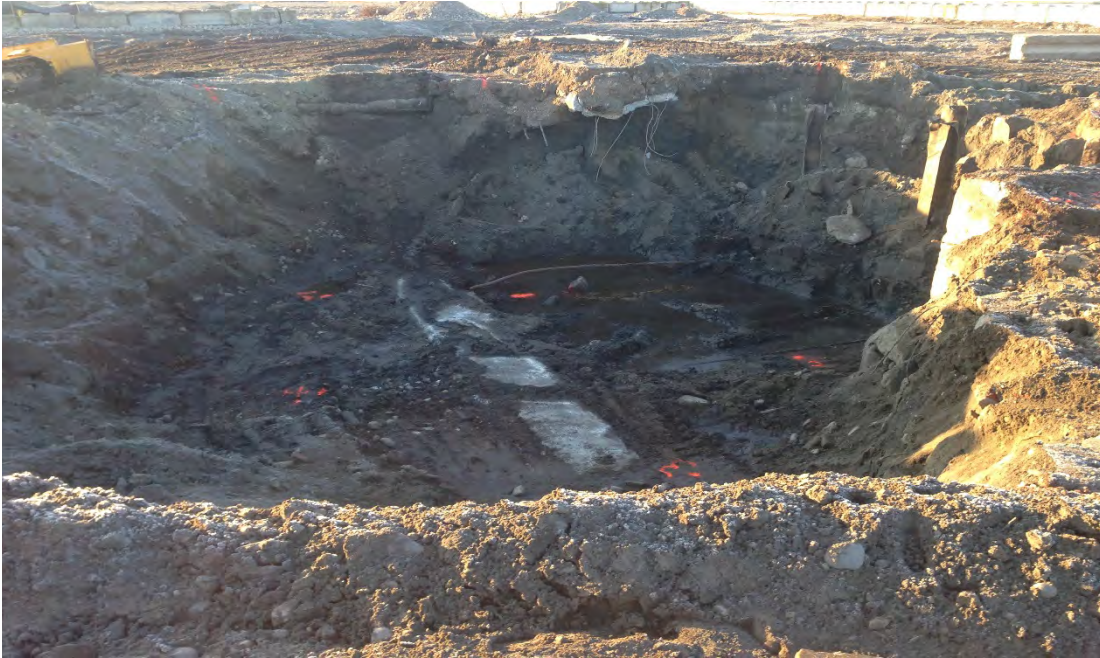
Photograph 27 – UST 70 excavation: looking south
