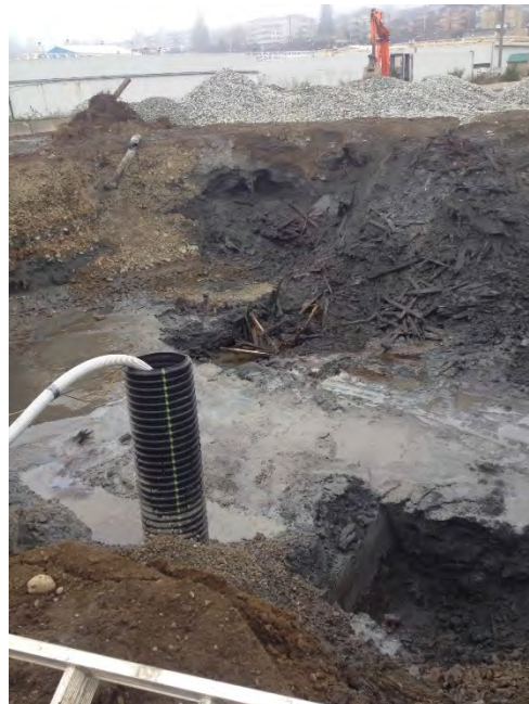
Photograph 14 – Naval Reserve Parcel UST excavation
