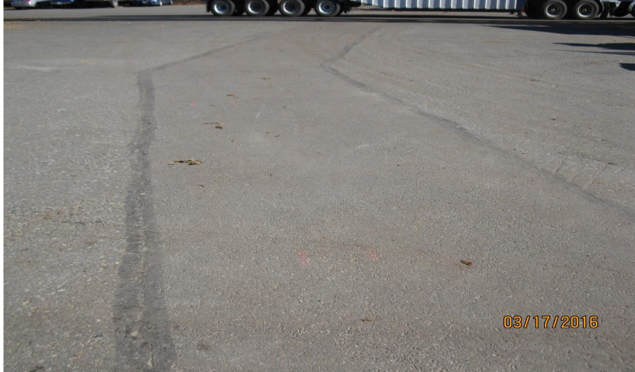
Photo 3: Edman Company Log Yard, Repaired Asphalt Cap– From South
