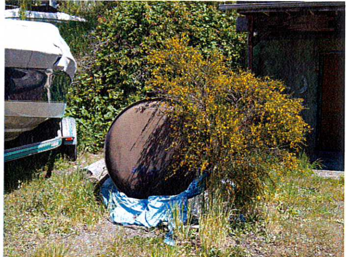
Photograph 4. Old waste oil storage tank located outside of the basement.
