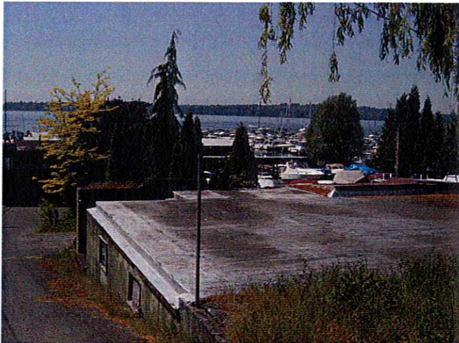
Photograph 3. Potential vent line protruding from the southern side of the 1950-vintage basement.
