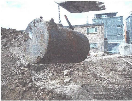
Photograph's above depict the 300 gallon heating oil UST and petroleum impacted soils from beneath the UST.
