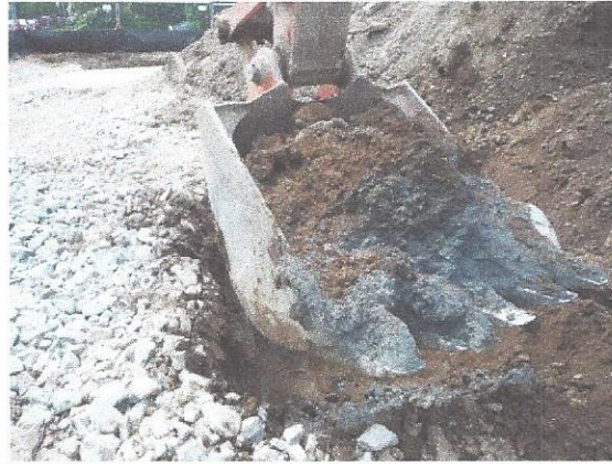
Photograph's above depict the 300 gallon heating oil UST and petroleum impacted soils from beneath the UST.
