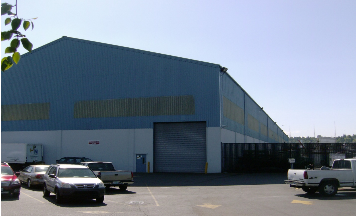
Photo 3: Warehouse – North End Looking Along the West Side (Fenced Area)
