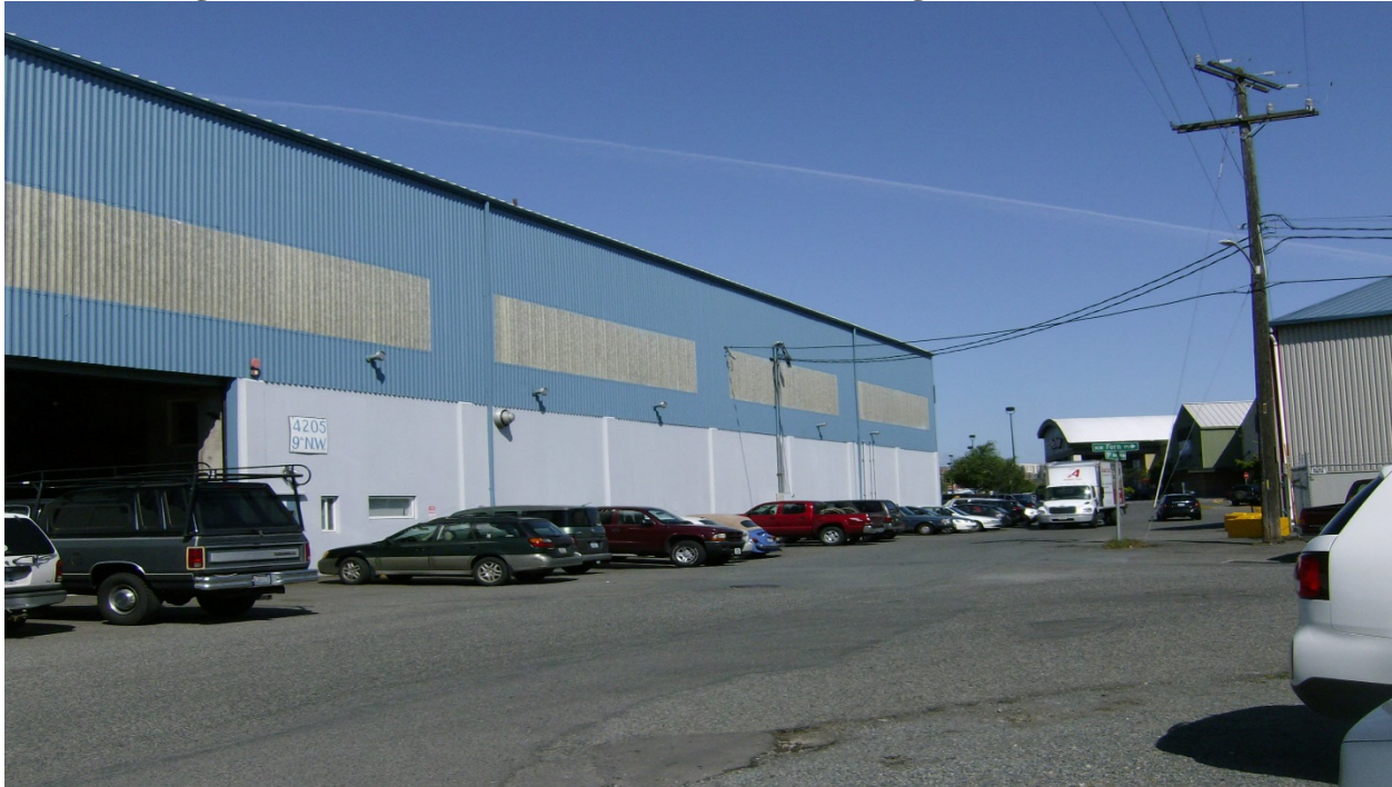
Photo 1: Ferguson Terminal Warehouse – East Side Looking North
