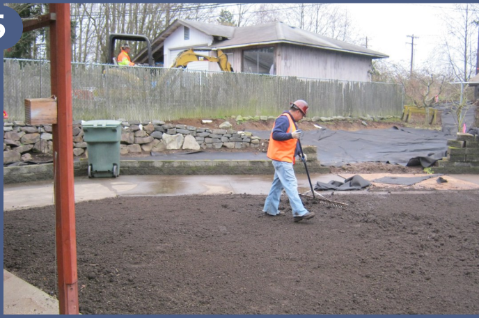
Top soil is applied.
