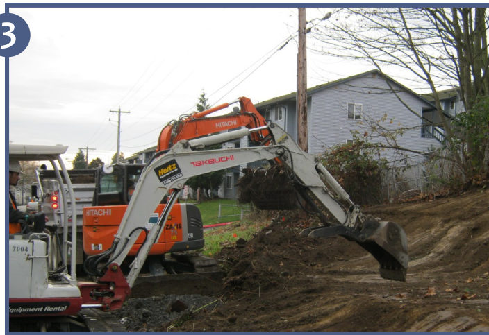
3 Contaminated soil is removed. Grass and plants are also removed.
