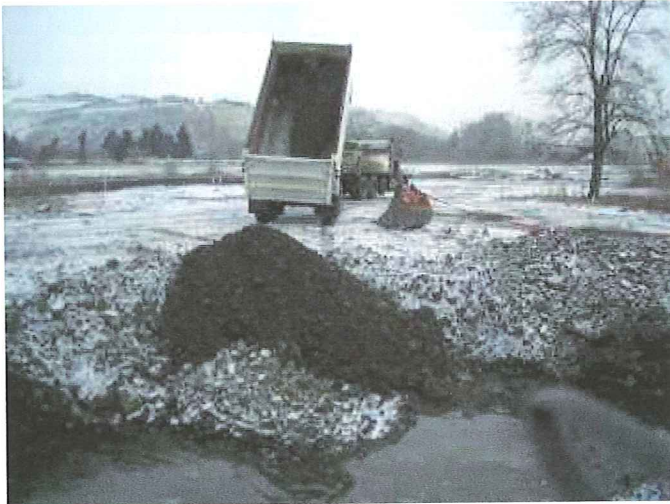
Photo 09 - Backfill placement - View south
