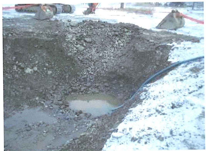
Photo 06 - Pumping water from east end of excavation
