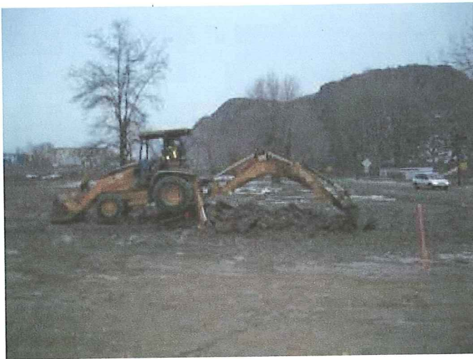
Photo 01 - Contaminated Soil Excavation - View east
