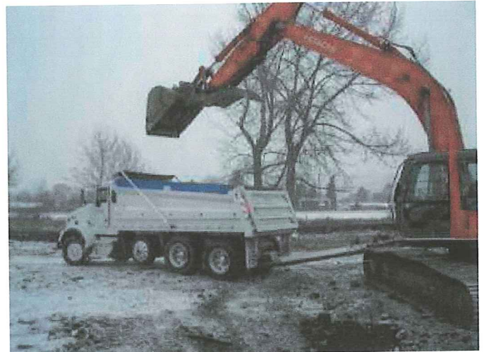
Photo 04 - Loading out contaminated soil
