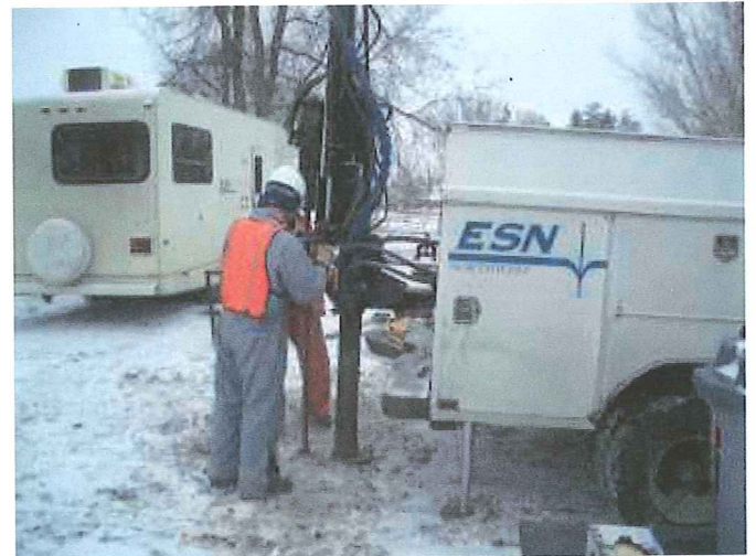
Photo 10 - Soil boring / well installation - B1/MW1
