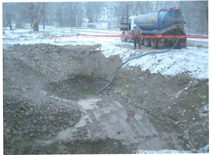
Photo 08 - Dewatering - South Excavation
