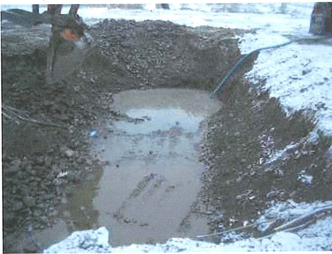
Photo 07 - Excavation Area - View Southwest
