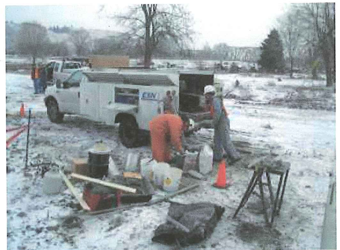
Photo 12 - Soil boring / well installation - B3/MW3
