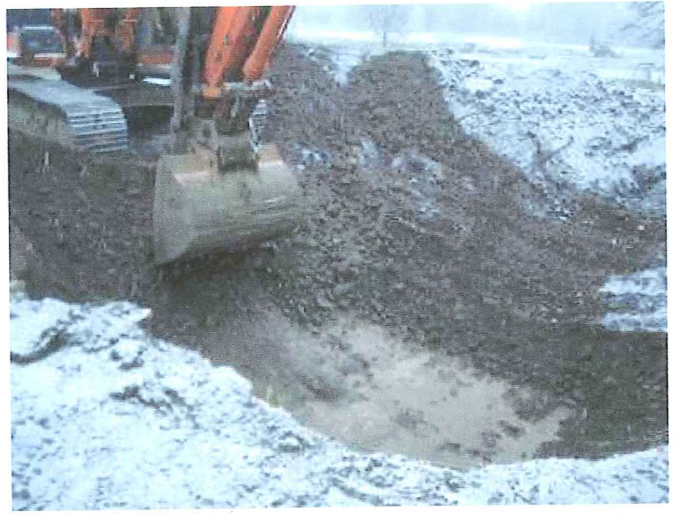
Photo 02 - Continued Contaminated Soil Excavation
