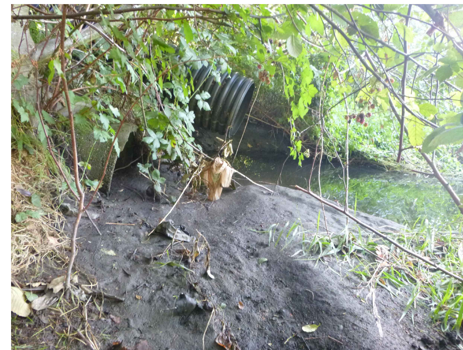
PHOTO D/CG09.1 EXISTING STORMWATER OUTFALL
