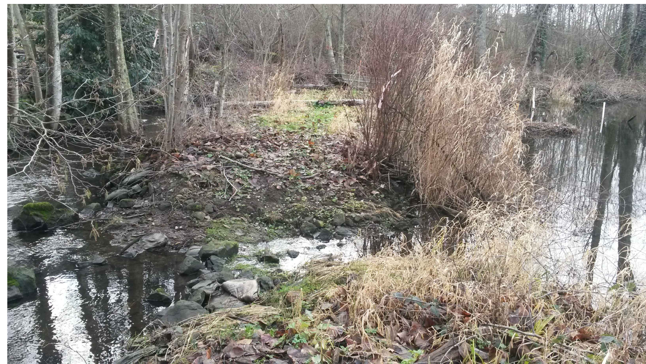
PHOTO C/CG09.1 EAST LAKE BERM AT CULVERT
