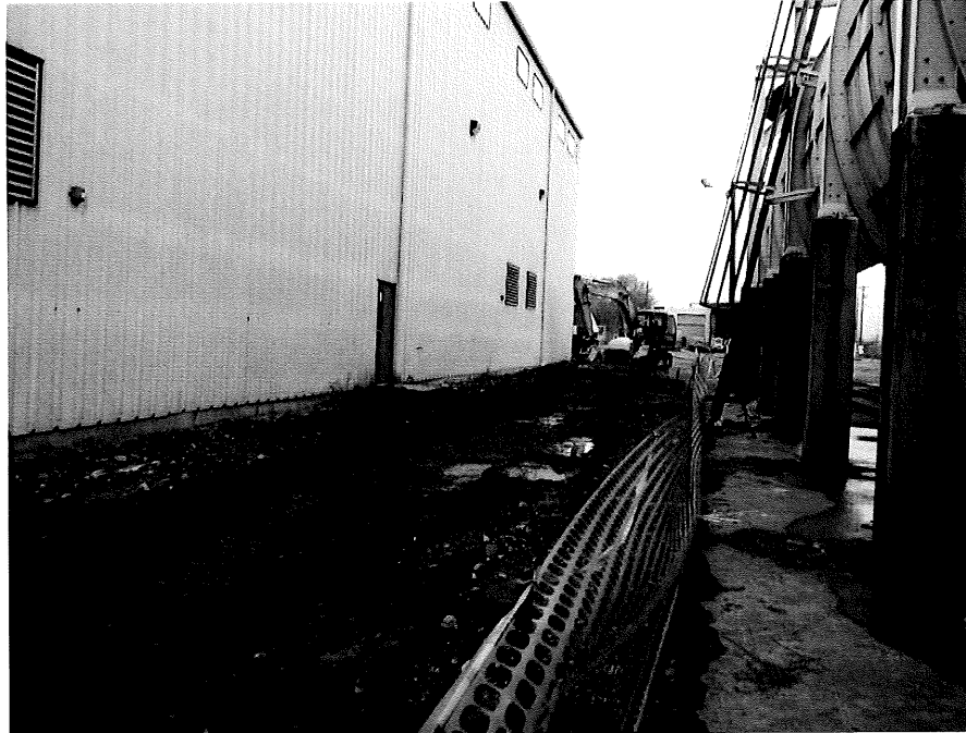
Photograph No. 9: View of the excavation area facing west.
