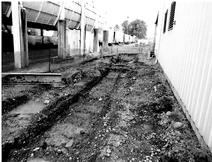
Photograph No. 8: View of the trench area backfilled, facing east.
