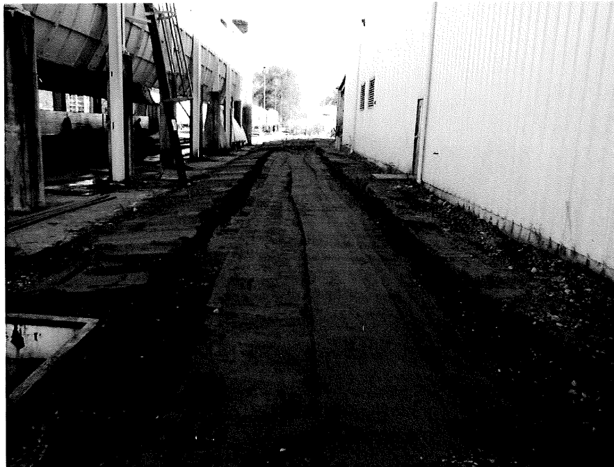
Photograph No. 10: View of the excavation area backfilled, compacted and ready for installation of new filter fabric and gravel railroad base.
