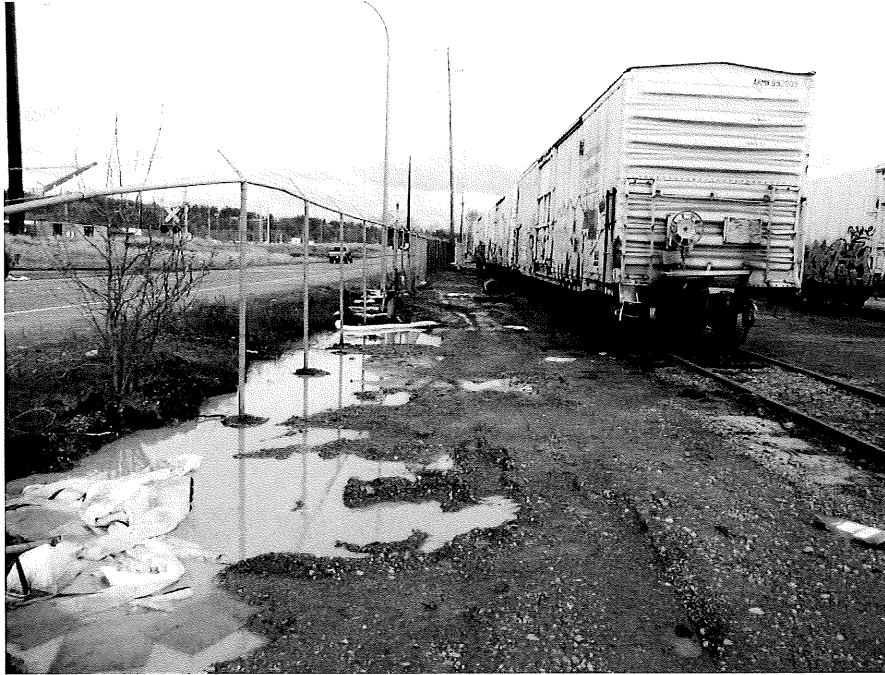
Photograph No. 1: View of the cleanup area with absorbent booms and pads, taken on February 19, 2014, facing east.
