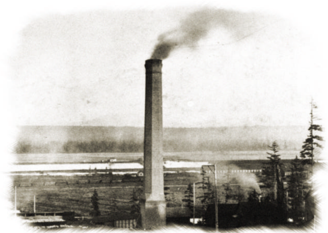
Puget Sound Reduction Works facility looking east. December 10, 1895. Duryee Collection. Courtesy of Everett Public Library
