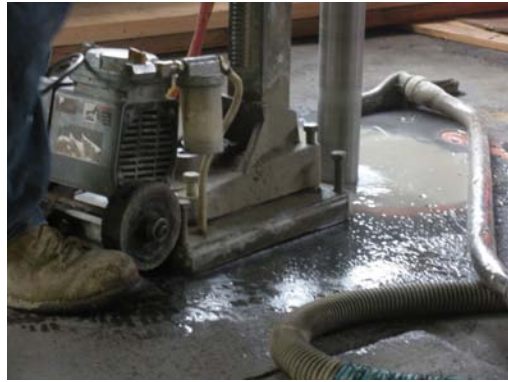
Photo 11 Top View Project Site Concrete Coring Typical Water was Vacuumed Off-Site Disposal
