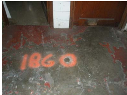
Photo 25 Top View Project Site Original Building Soil Sample 1BG Background #1 Sacrete Top Seal Typical
