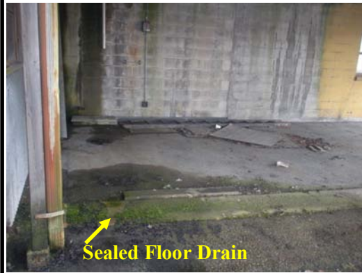
Photo 6 Facing Northwest Project Site Third Addition Pole Roof Sealed Floor Drain Soils 20 to 23
