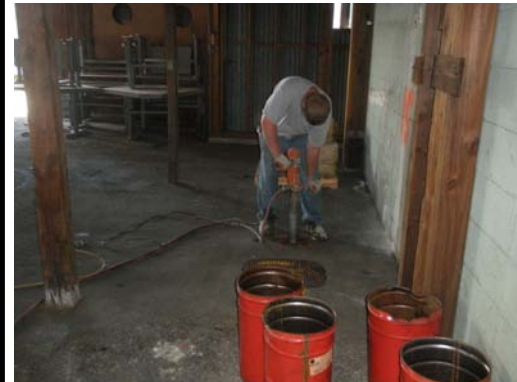
Photo 12 Facing West Project Site Second Addition Concrete Coring Typical Water was Vacuumed Off-Site Disposal
