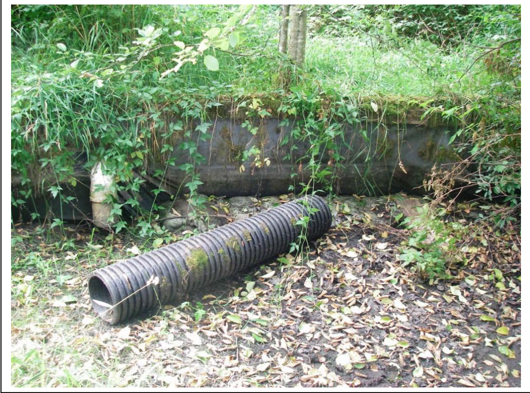
Dam 1 at south end of project site
