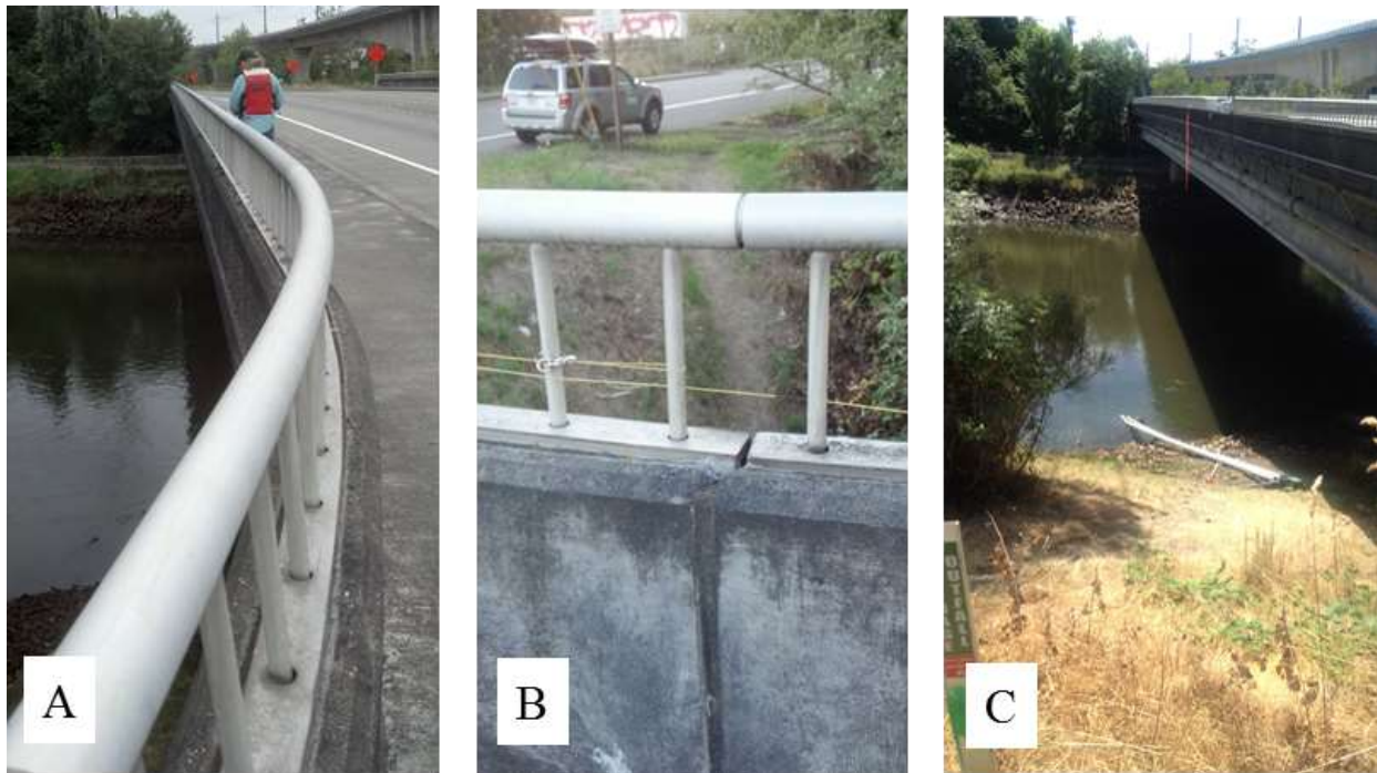
Figure 5. Site photographs of the downstream station (USGS 12113415) including (A) the pedestrian sidewalk, (B) off-road parking and bank access, and (C) shoreline access.
