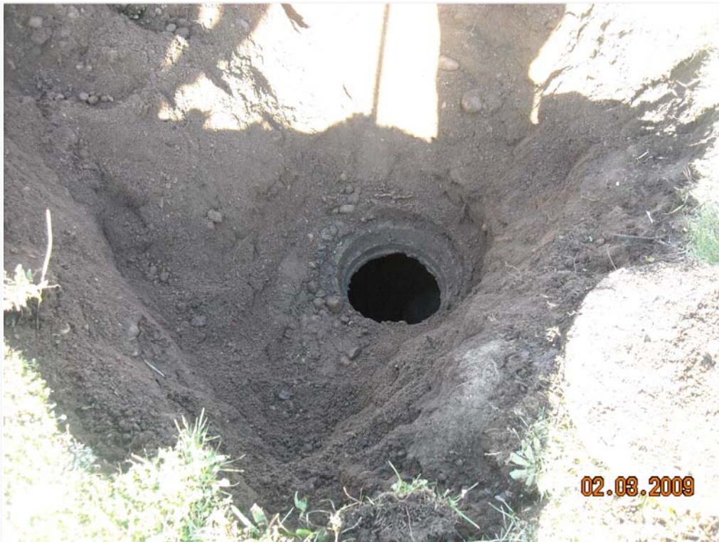
Photo 3. Small access lid into top of drywell.
