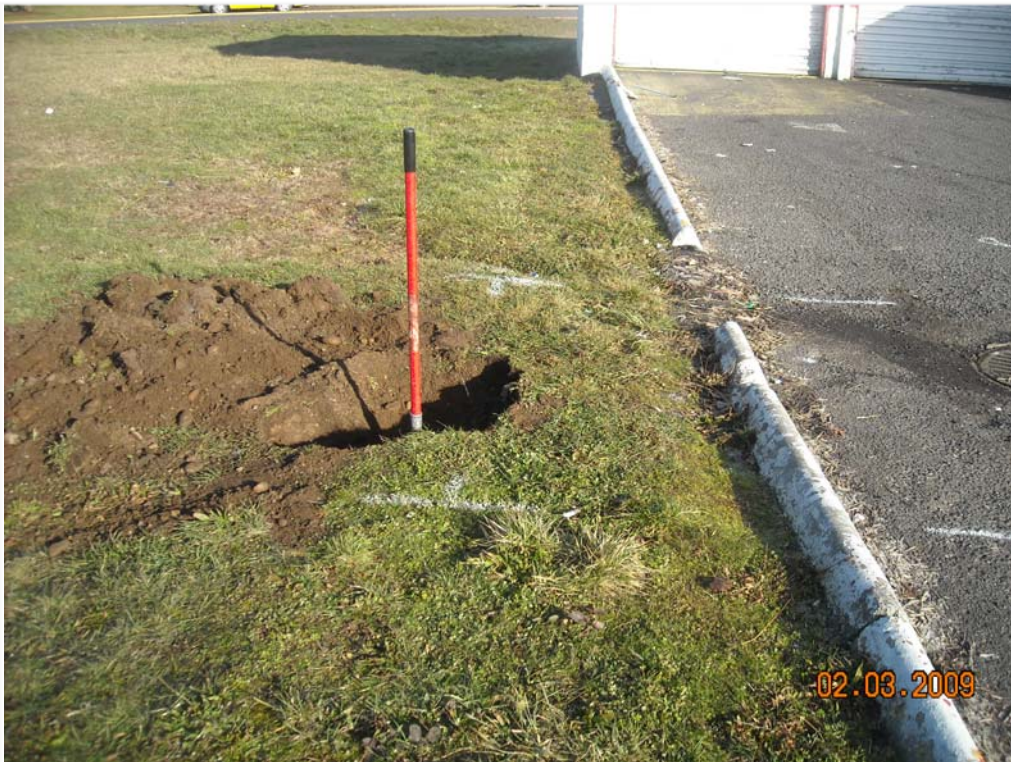
Photo 1: Attempt to unearth top of drywell with hand tools (e.g. shovel)
