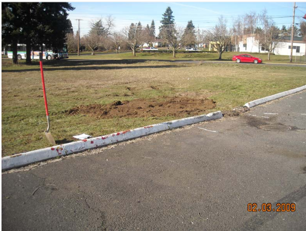
Photo 6. After covering of drywell, prior to leaving site.
