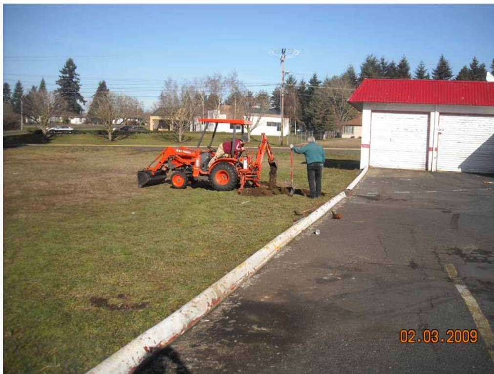
Photo 2: Small backhoe brought in to complete excavation.
