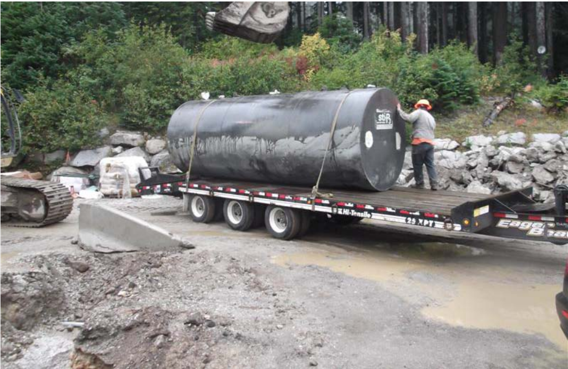
4,000-gallon gasoline UST after removal.
