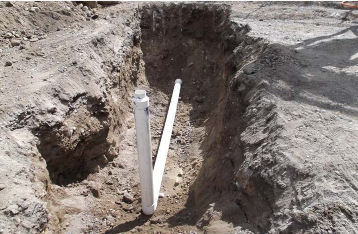
Construction of reinfiltration trench.
