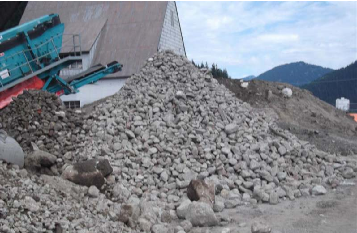
Stockpile of coarse material after passing through screener.
