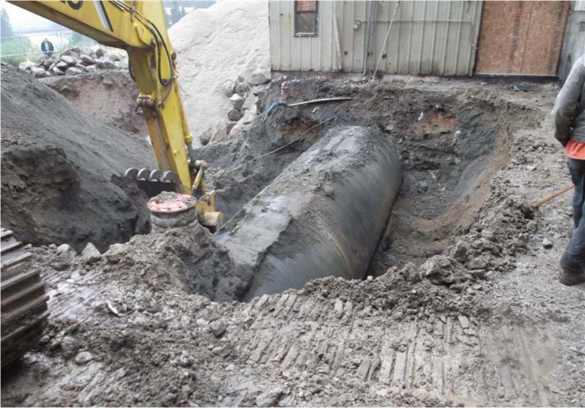
West to east view of 10,000-gallon diesel UST prior to removal.
