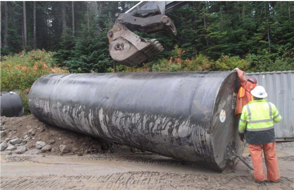
10,000-gallon diesel UST after removal.
