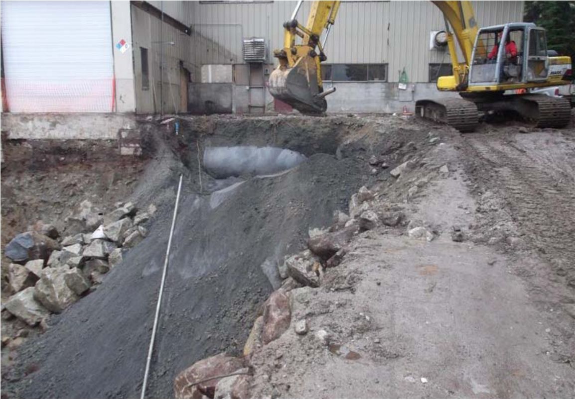
North to south view of 4,000-gallon gasoline UST prior to removal.
