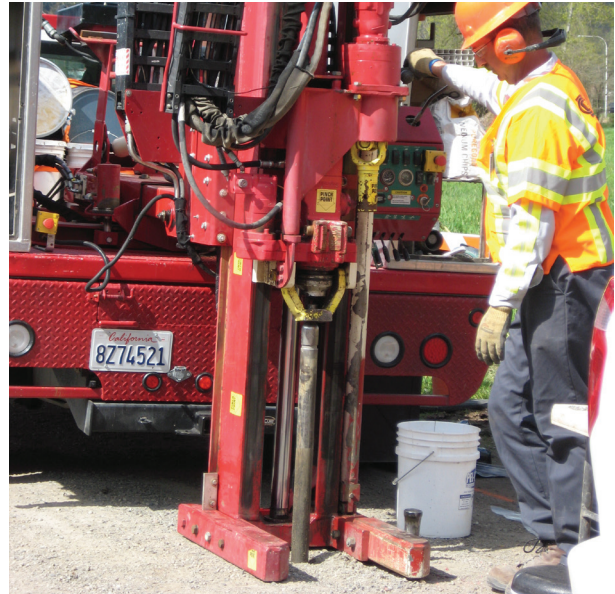
Drilling for groundwater samples in northeast Algona.
