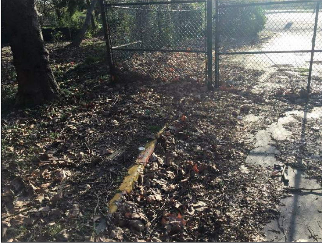
Photo 01 (LLA- L01): Painted Concrete Curb Near Property Entrance. (3/25/16)
