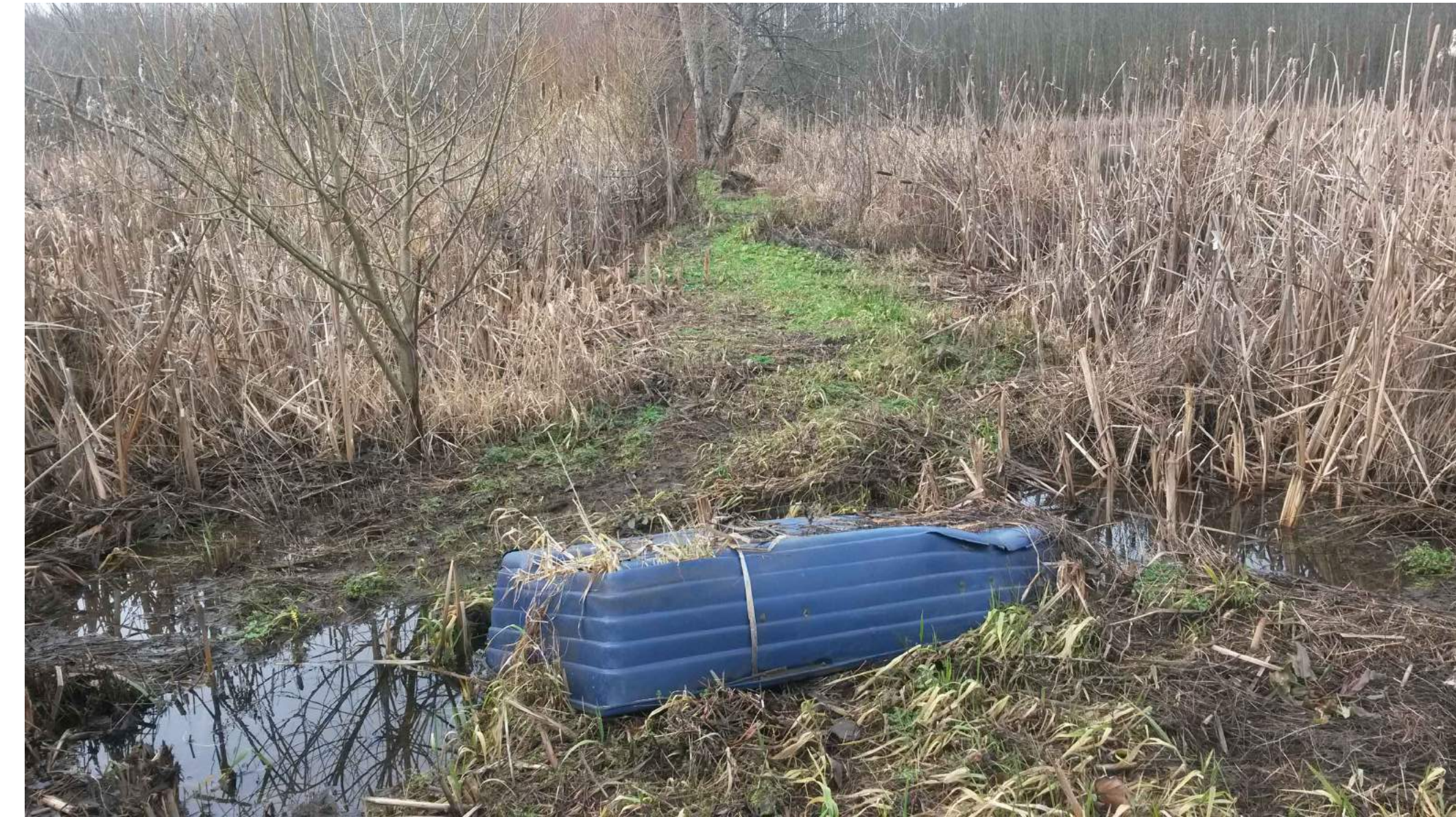
PHOTO B/CG09.1 SOUTH LAKE BERM LOW SPOT
