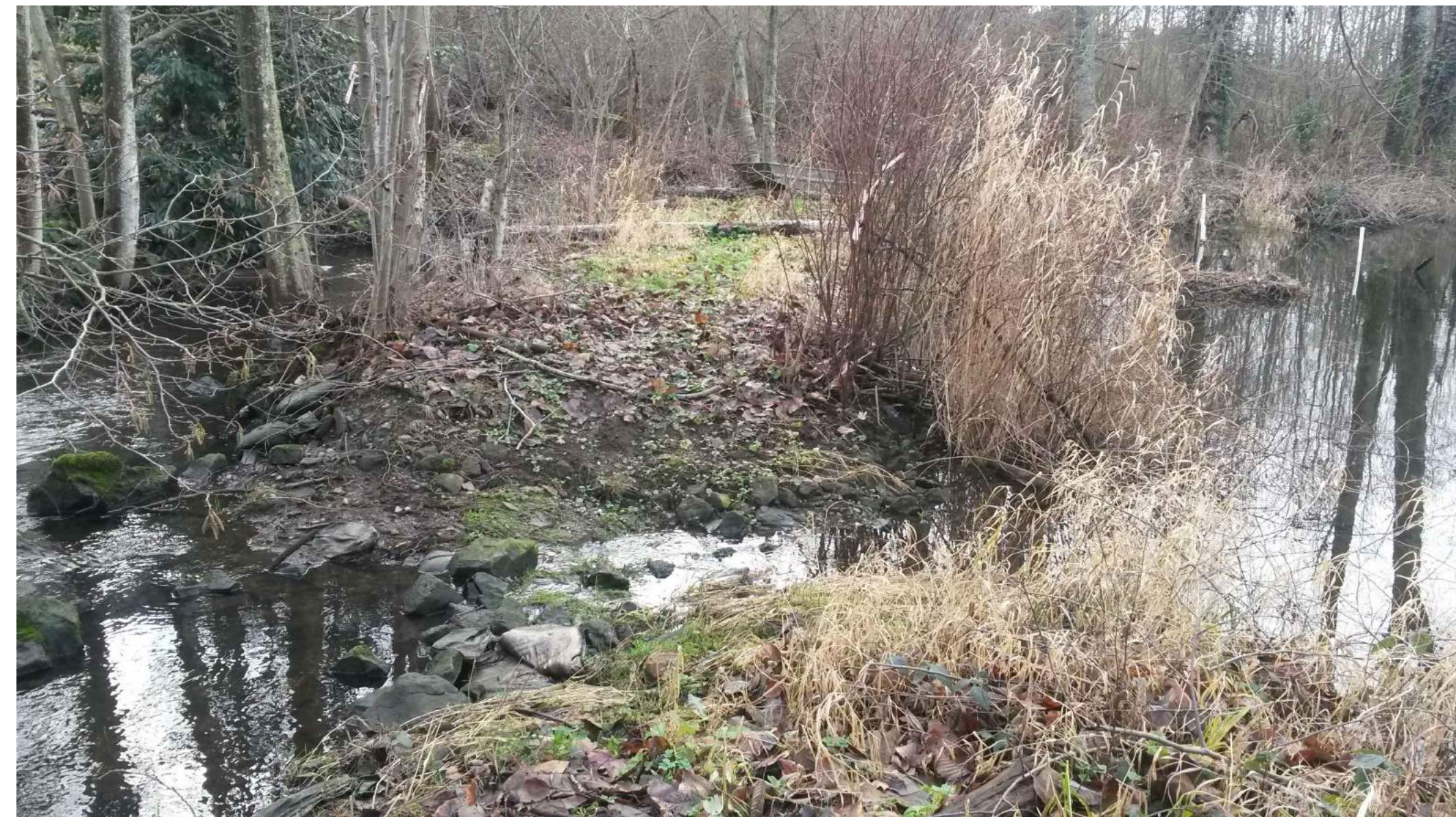
PHOTO C/CG09.1 EAST LAKE BERM AT CULVERT
