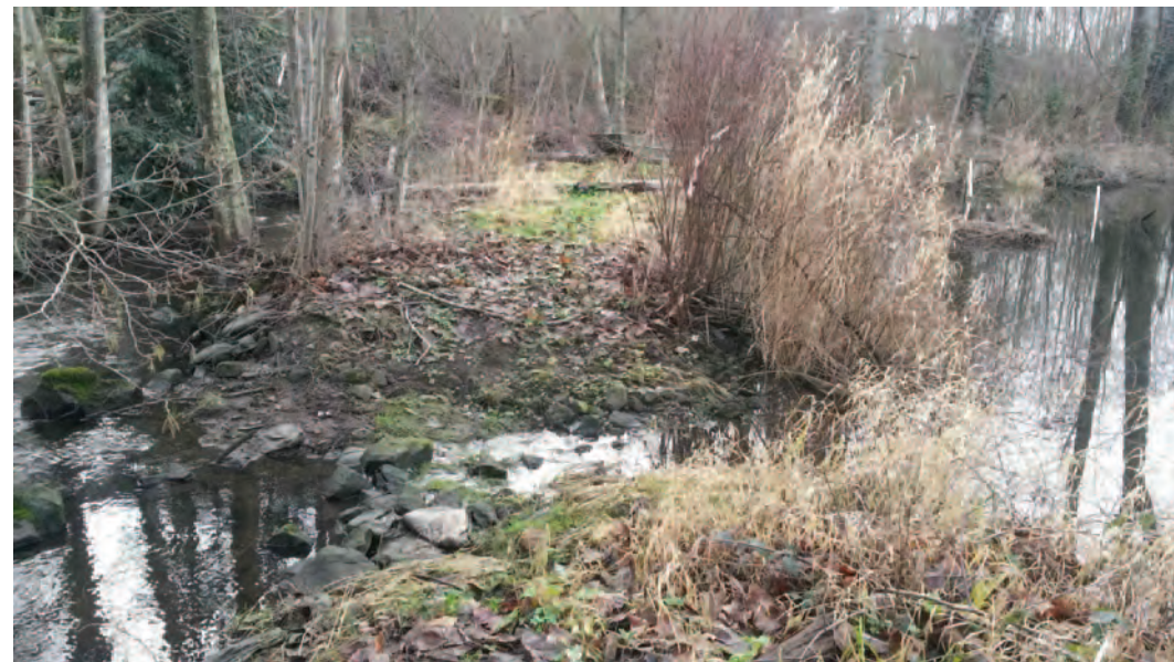
PHOTO CG09.1 C - EAST LAKE BERM AT CULVERT
