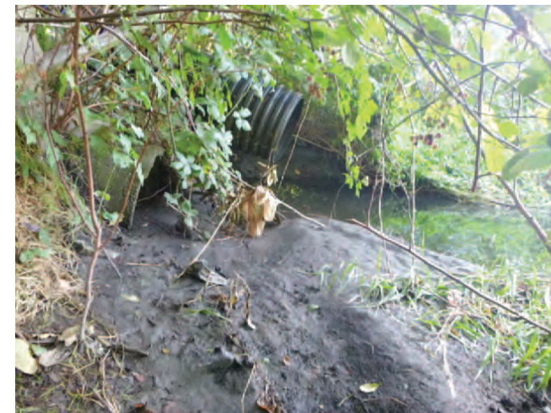
PHOTO CG09.1 D - EXISTING STORMWATER OUTFALL
