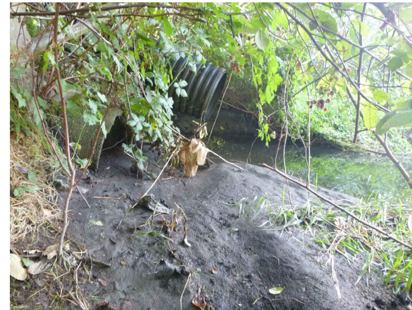
PHOTO D/CG09.1 EXISTING STORMWATER OUTFALL
