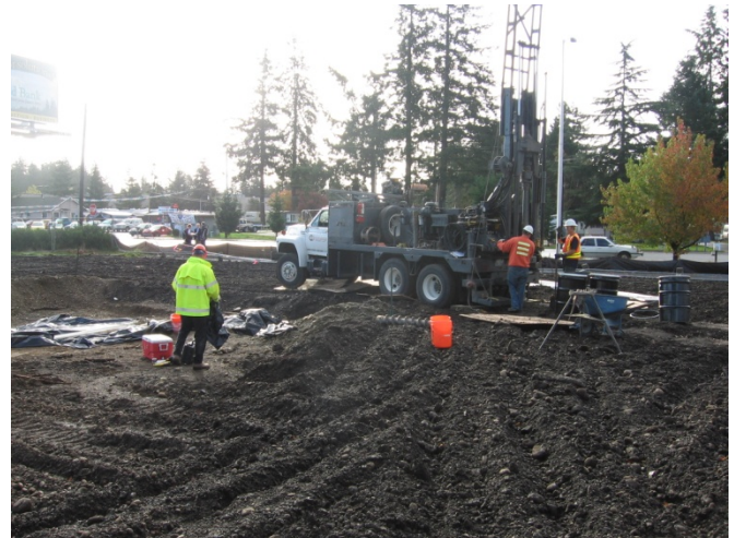
Photograph 12. Monitoring well installation
