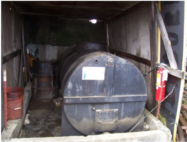
Photograph 3. Former aboveground storage tank
