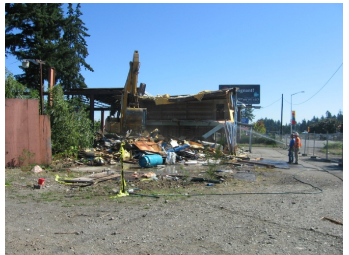
Photograph 6. Building demolition activities
