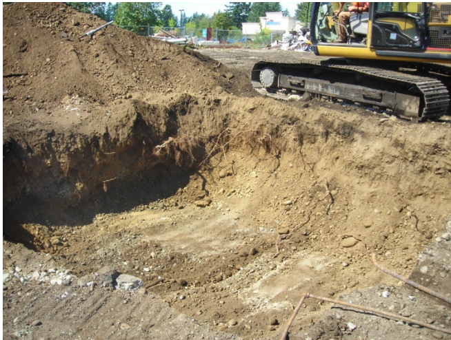
Photograph 9. Underground storage tank excavation
