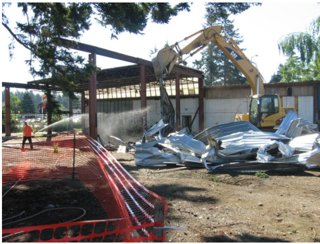
Photograph 7. Canopy demolition activities
