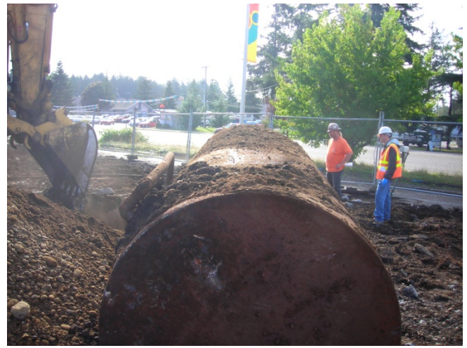
Photograph 8. Underground storage tank pull
