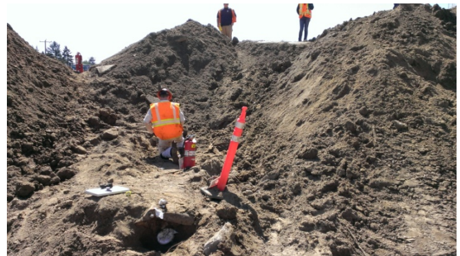
Photograph 4. Marine Chemist inerting UST07.
