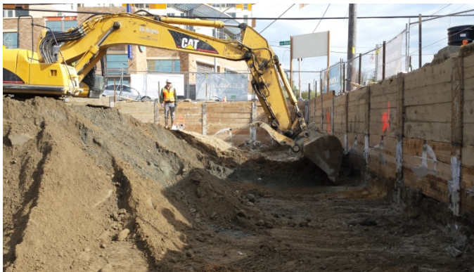
Photograph 5. Excavating east wall of the Property to approximately 10 feet bgs.
