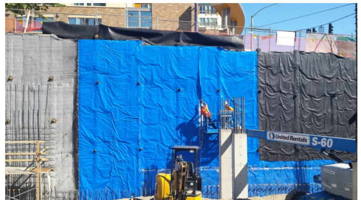
Photograph 18. Application of the protective fabric over the Liquid Boot.
