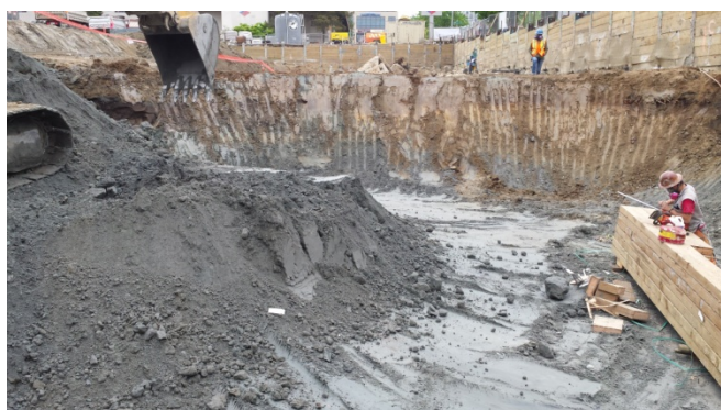
Photograph 9. Excavating to approximately 15 feet below ground surface. Respirators required by all personnel working within the contaminated area.
