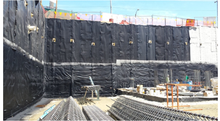
Photograph 14. Completed application of Liquid Boot on basement level.
