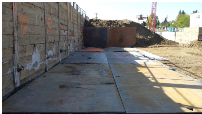
Photograph 7. Plastic and metal plates placed south of the Property for a loading dock for contaminated soil.
