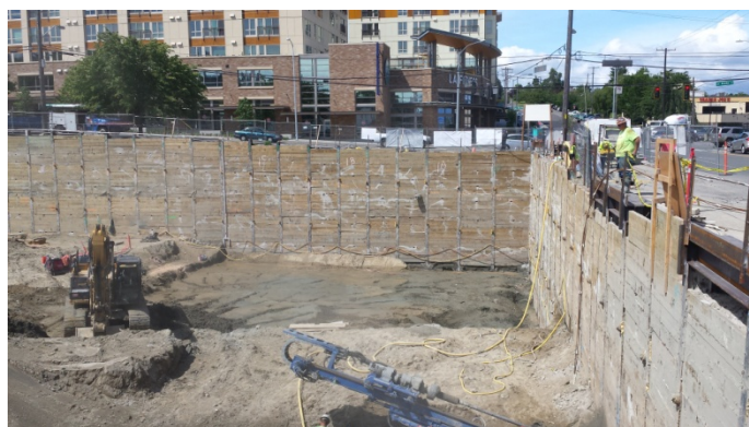
Photograph 12. Final extent of the petroleum contamination excavation at the Property.
