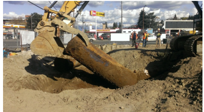
Photograph 2. Removing UST06.
