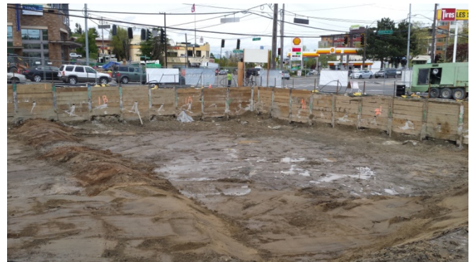
Photograph 6. The Property excavated to 10 feet bgs.
