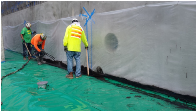
Photograph 21. Application of Liquid Boot layer up against the sidewall.
