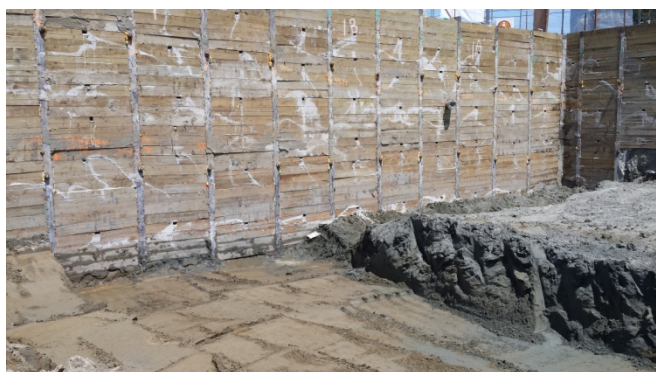
Photograph 9. Excavating to approximately 15 feet below ground surface. Respirators required by all personnel working within the contaminated area.
