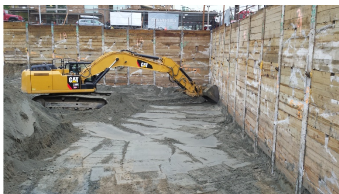
Photograph 10. Excavating down to approximately 20 feet below ground surface.
