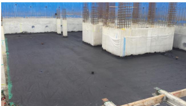
Photograph 23. Completed Liquid Boot installation on the floor of the Property.
