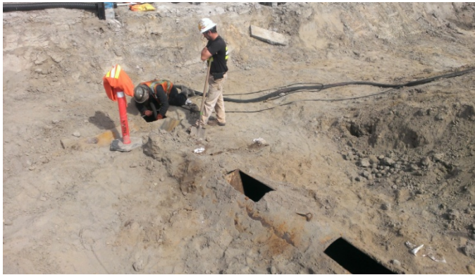
Photograph 1. Marine Vacuum Services emptying UST05 and UST06.
