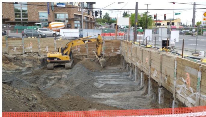
Photograph 8. Excavating down to approximately 15 feet below ground surface, view looking north.
