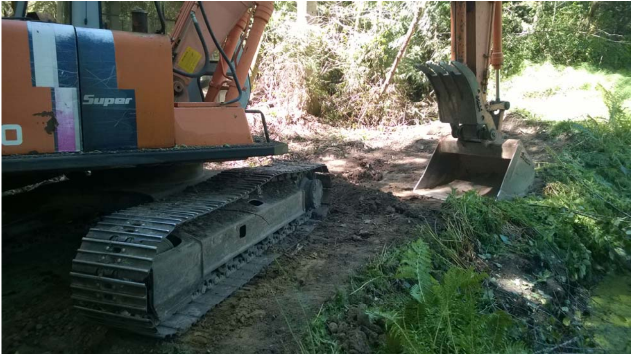
Photo 5: Beginning of Excavation of Southern Area
