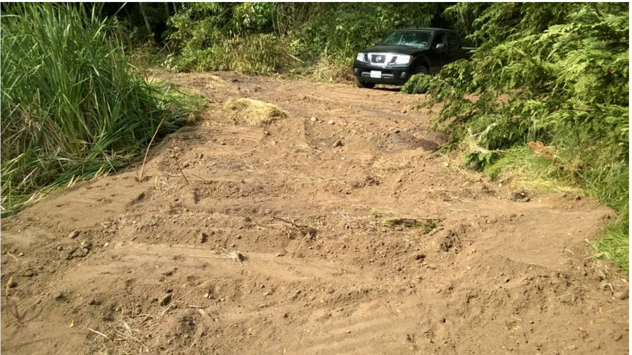
Photo 12: Backfilled Northern Area Looking West
