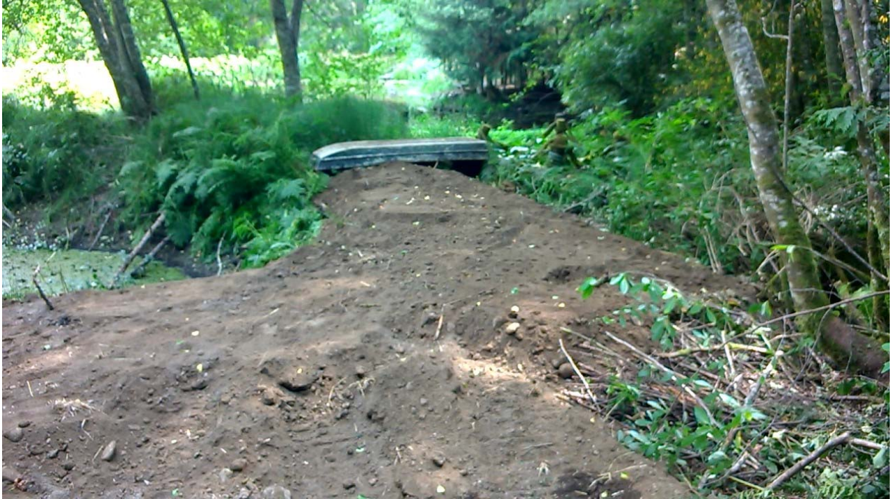
Photo 9: Backfilled Southern Area Looking North
