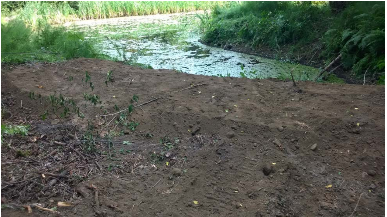
Photo 10: Backfilled Southern Area Looking East
