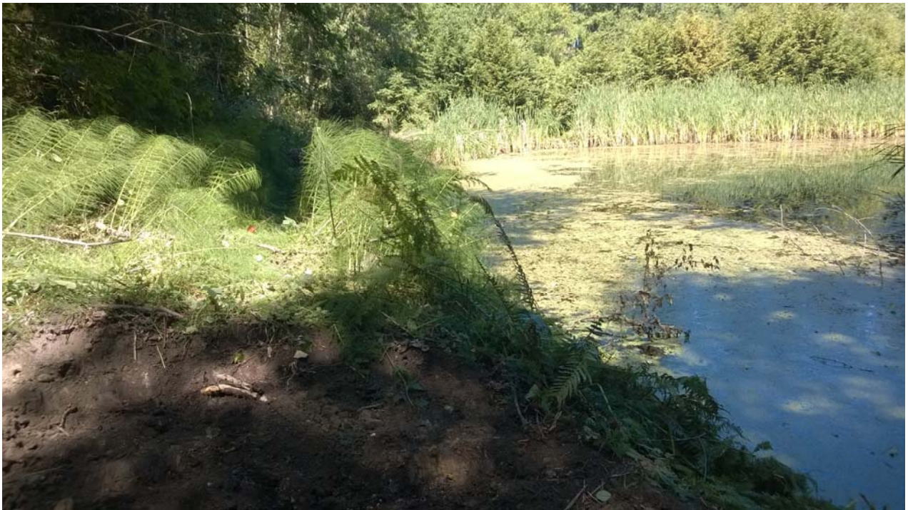
Photo 6: Southern Limit of Excavation in Southern Area
