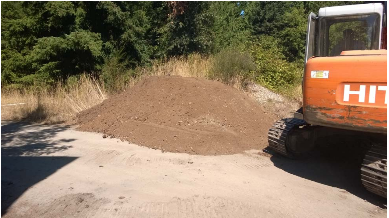
Photo 8: Imported Backfill Pile
