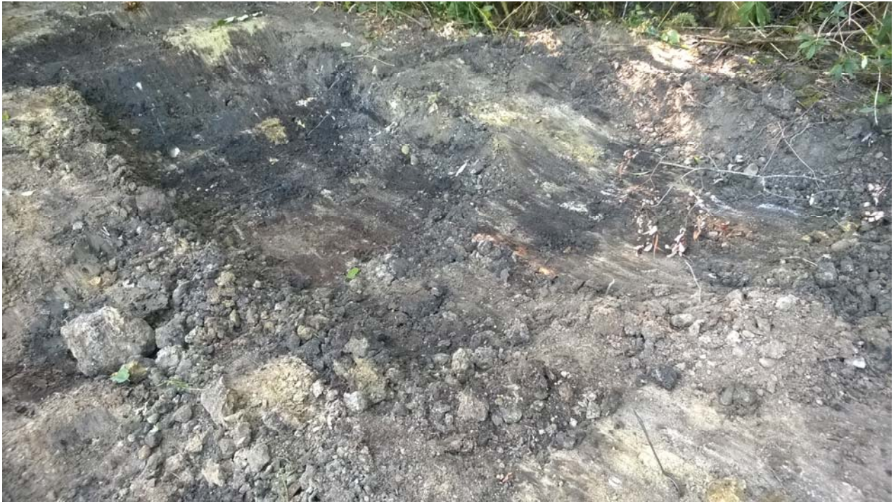
Photo 7: Base of Excavation in Middle Area where confirmation samples were collected and initially failed. This area was re-excavated.
