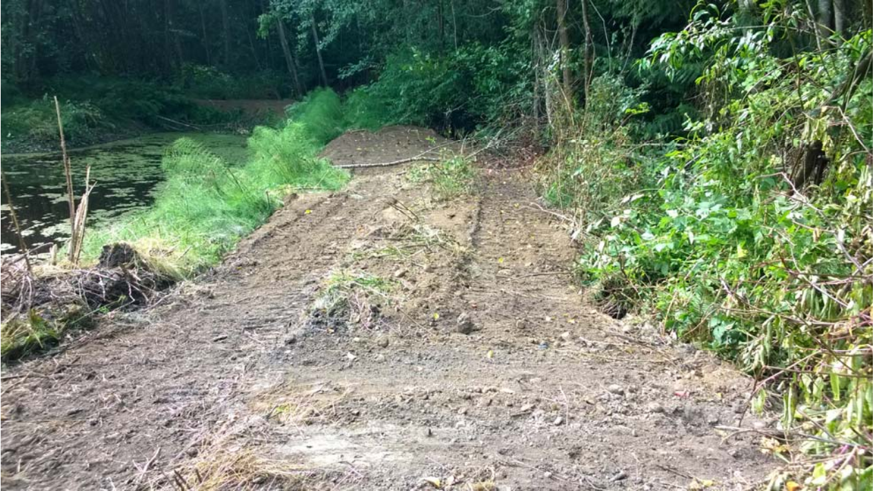
Photo 11: Backfilled Middle Area Looking North
