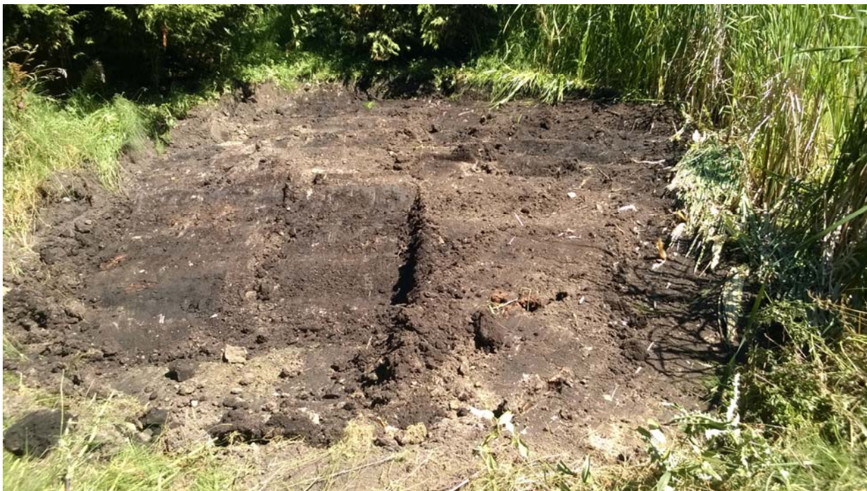
Photo 1: Northern Excavation Area
