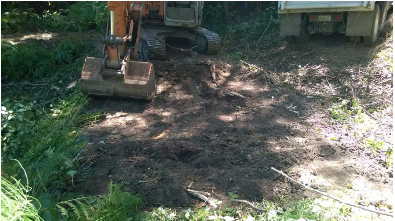
Photo 4: Digging Out Southern Area
