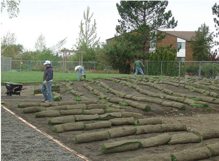
Figure 1. Skyline Montessori, Tacoma: Sod being laid over clean soil.
