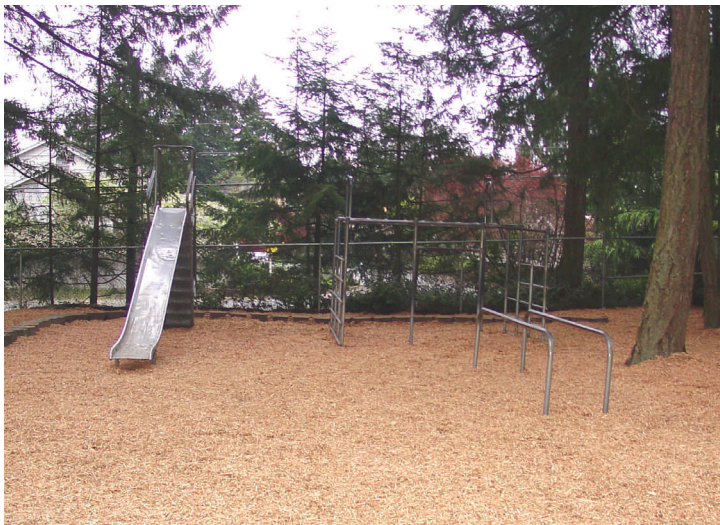
Figure 2. Heritage Christian School, University Place: A new wood chip play surface covers an area where polluted soils were removed.
