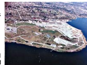
Figure 10: Construction of NOAA Campus 1981-82 (JPG)
